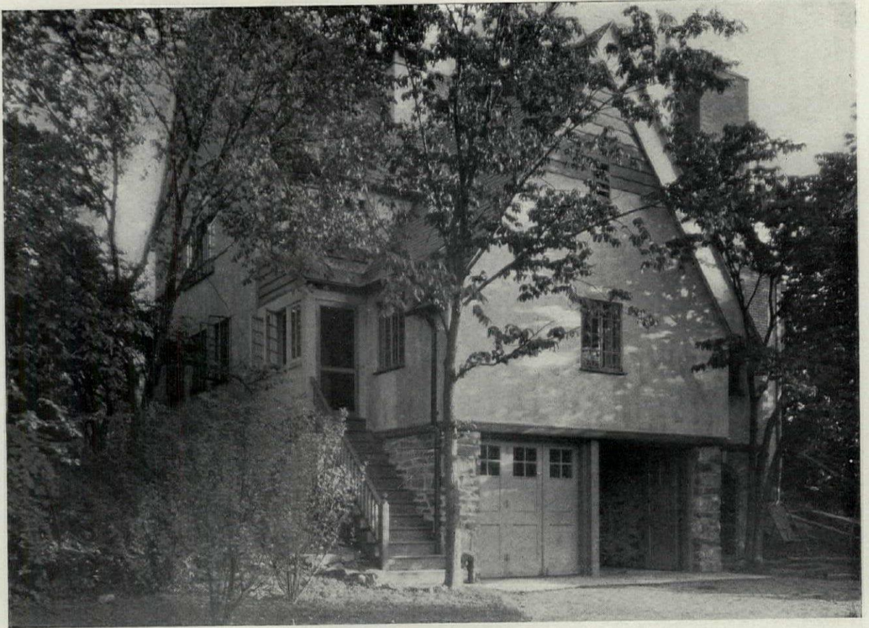
SERVICE ENTRANCE AND GARAGE
