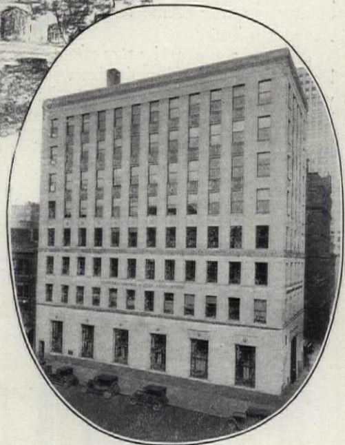
A recent Duraflex-A Installation in Detroit, Michigan STANDARD SAVINGS & LOAN ASSOCIATION BUILDING GEORGE D. MASON & CO., Architects W. E. Wood Co., Contractors
