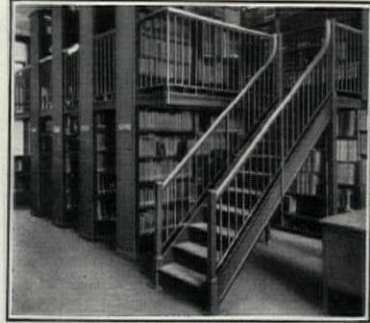
Art Metal two-story library stack in the Federal Reserve Bank in Philadelphia. Bunting & Shrigley, architects.
