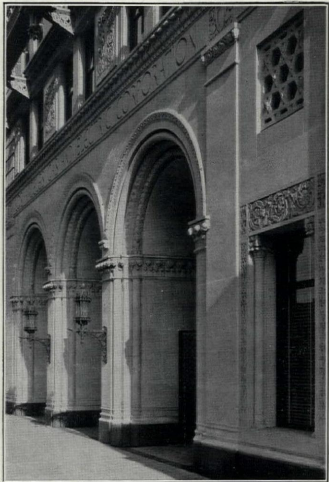
Los Angeles Gas & Electric Corporation Bldg., Los Angeles, Calif. J. B. & Donald Parkinson, Architects.
