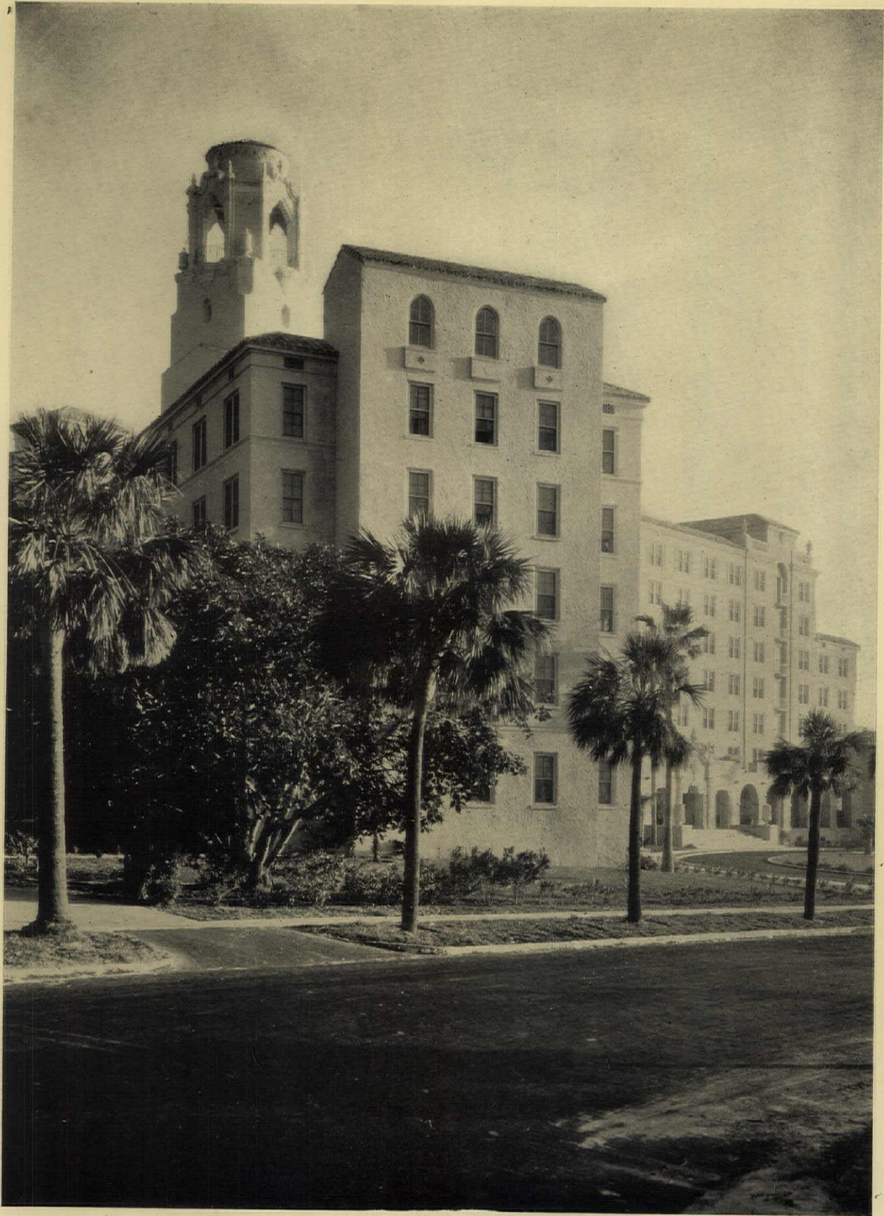
SOUTHERN WING VINOY PARK HOTEL, ST. PETERSBURG, FLA. HENRY L. TAYLOR, ARCHITECT
