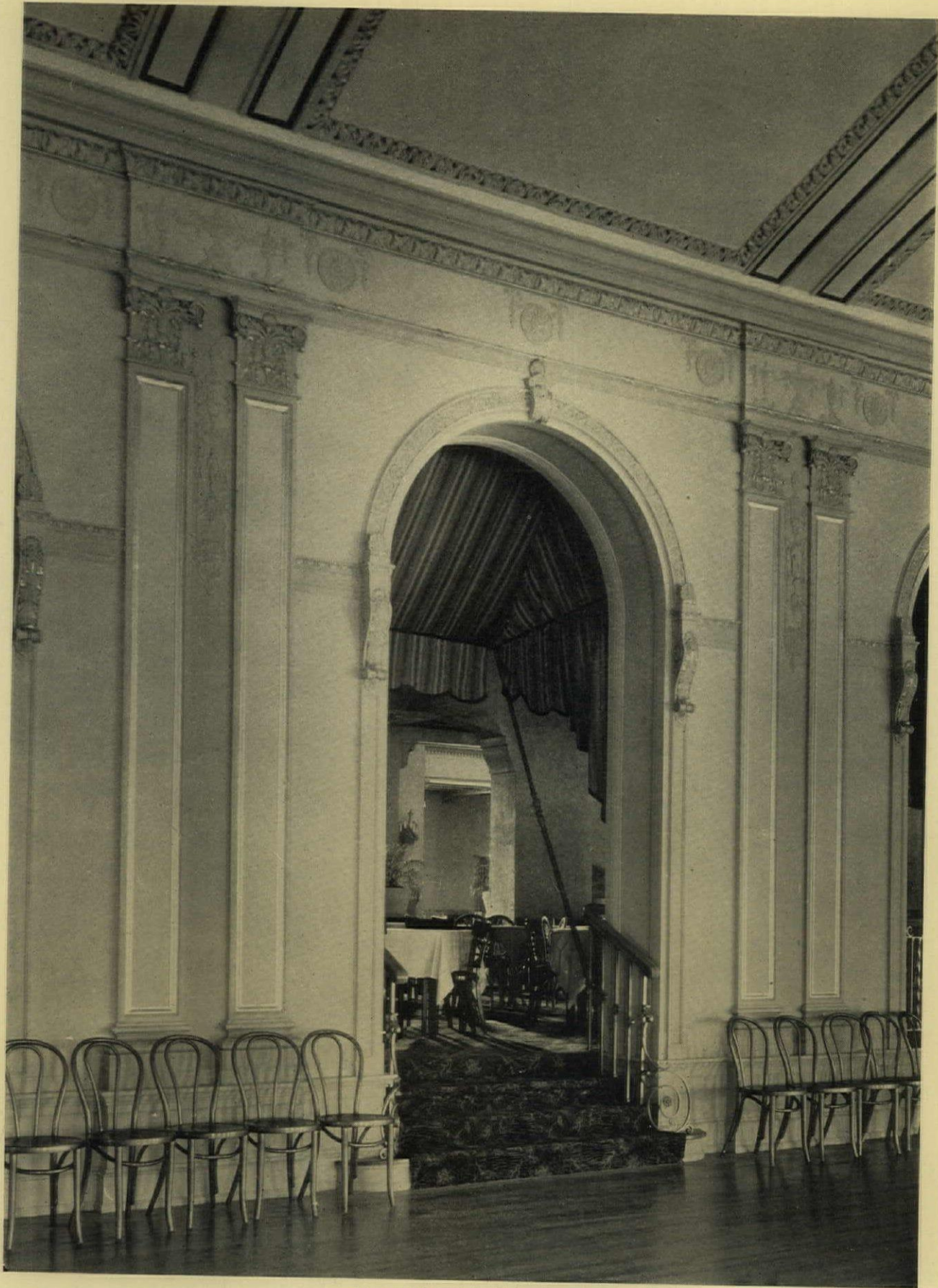
ENTRANCE TO BALL ROOM VINOY PARK HOTEL, ST. PETERSBURG, FLA. HENRY L. TAYLOR, ARCHITECT
