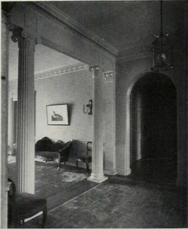
Detail in Main Hall
