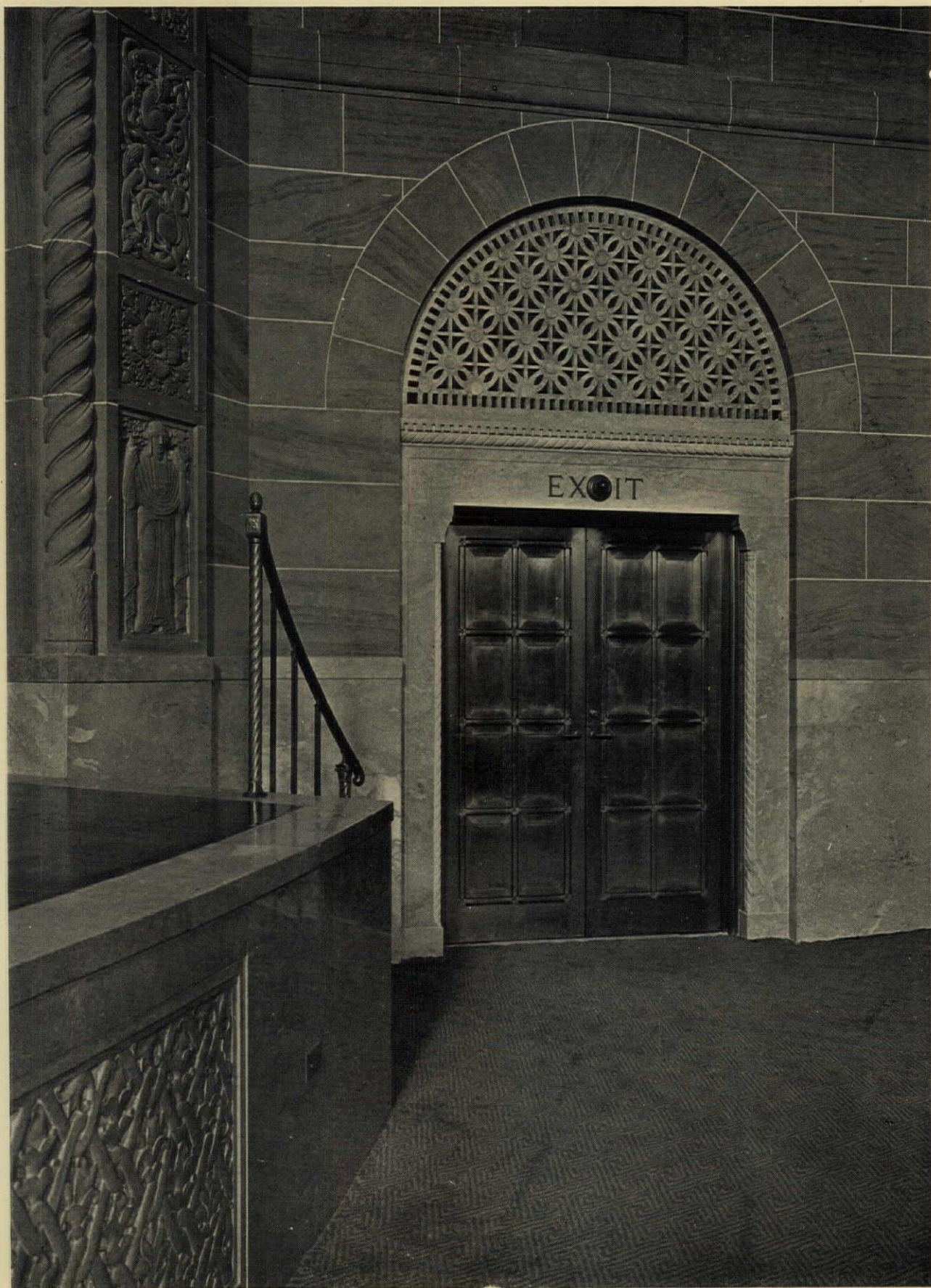
CORNER OF STAGE IN AUDITORIUM NEW YORK ACADEMY OF MEDICINE YORK & SAWYER, ARCHITECTS
