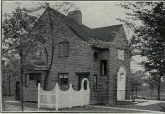
Residence of H. I. Glazier, Asst. Sales Mgr., General Fireproofing Co., Youngstown, Ohio. Built to First Prize Plan of Weyerhaeuser Lumber Co. Competition 1926. Insulated with Cabot's Quilt. Exterior Walls, Cabot's Stained Shingles. Exterior Trim finished with Cabot's Old Virginia White Collopakes. Johnson & Carlson, Youngstown, Ohio, General Contractors.
