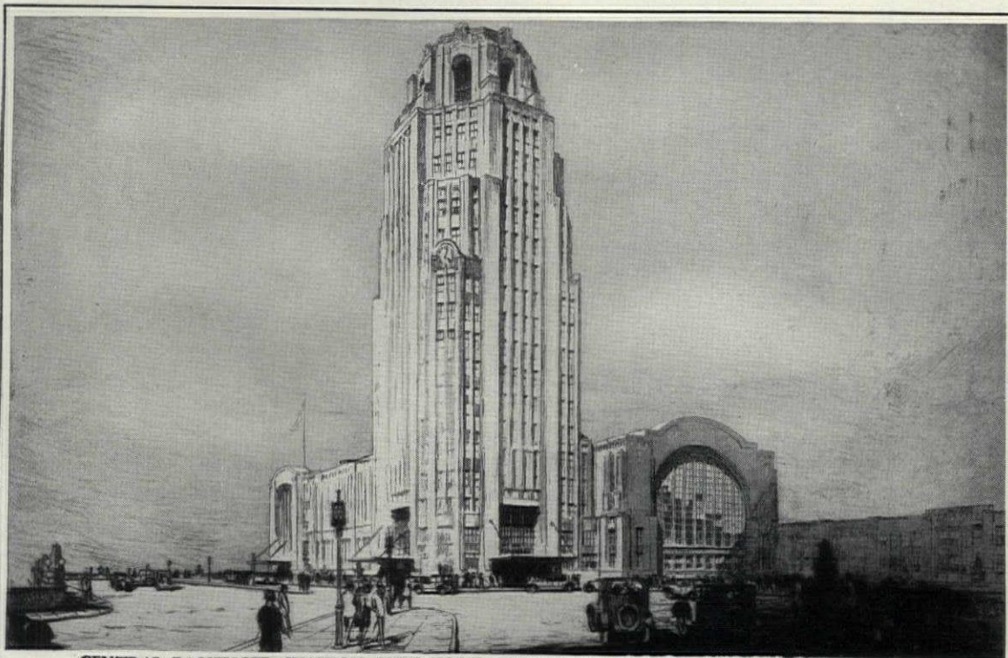
CENTRAL PASSENGER STATION, NEW YORK CENTRAL RAILROAD COMPANY, BUFFALO, N. Y. Architect and Engineer—Alfred Fellsheimer & Stuart Wagner, New York City; Heating Contractor—William E. Shattuck Co., Buffalo, N. Y.; Fan Equipment—Buffalo Forge Company. 12,022 square feet of VENTO.
