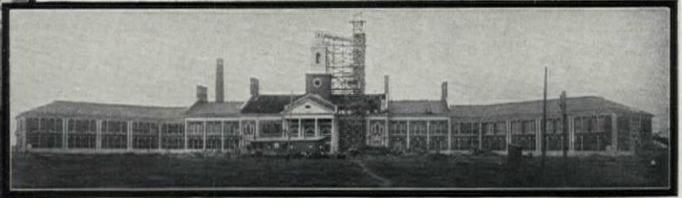
Grosse Pointe High School Grosse Pointe, Michigan Architect, George J. Haas
