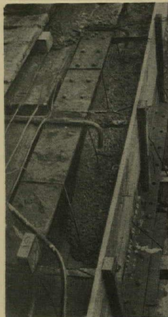
The beams were deep and wrapped with wire mesh. The extremely narrow space between the steel and framework at the corners would have made it almost impossible to get plain concrete well down around the under side of the beams. Here is where the added workability imparted by Celite proved especially valuable.
