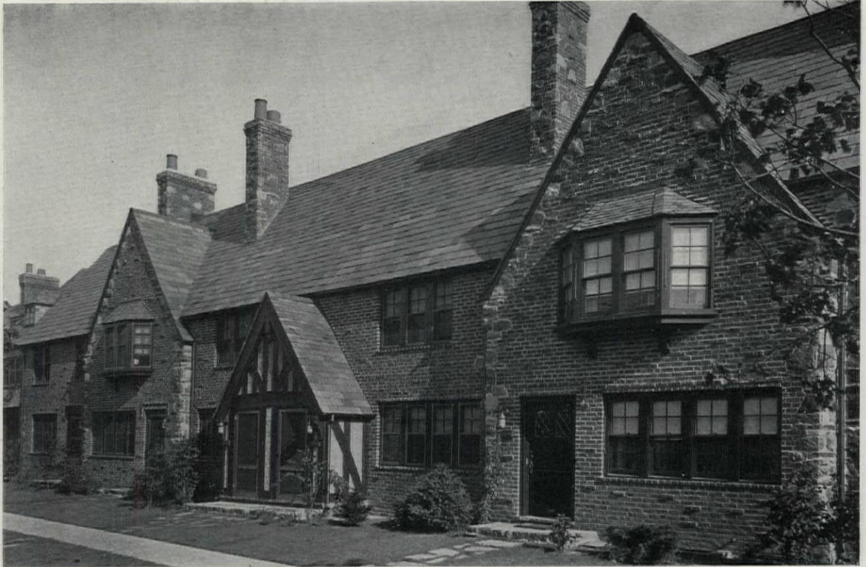
Interesting Grouping and Texture at Forest Close Robert Tappan, Architect
