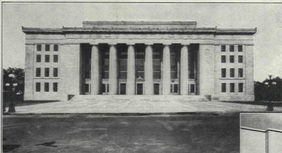
Wyandotte County Court House, Kansas City, Kansas. Architects—Wight and Wight; General Contractor—Swenson Construction Co.; Plumbers installing Youngstown Pipe—Interstate Heating & Plumbing Co., all of Kansas City, Mo.
