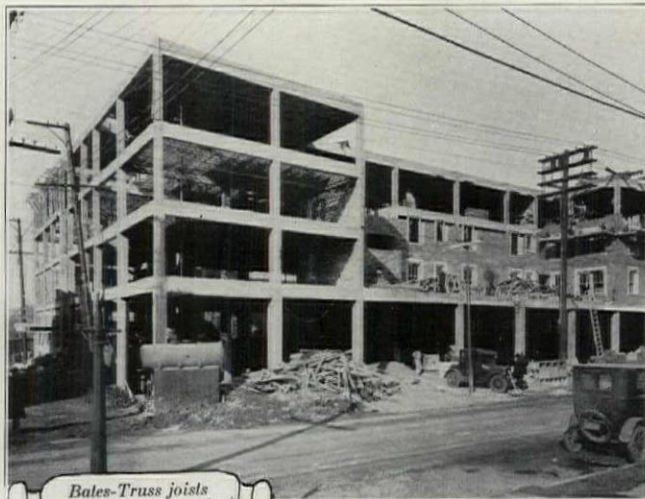
Bates-Truss joists in concrete construction St. Louis Mo.
