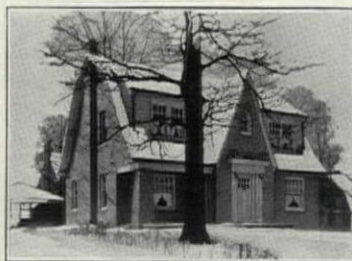
Masonite Insulating Lath used as plaster base. Owner, James Wagstaff, Youngstown, O. Contractor, Harry Garde, Cleveland
