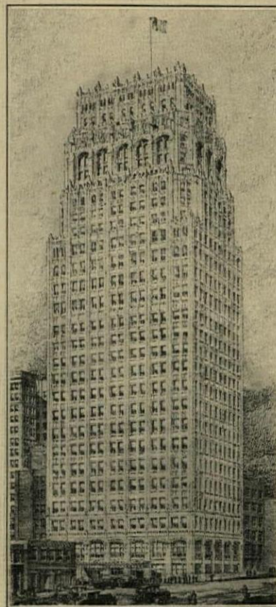
BELL TELEPHONE COMPANY BUILDING KANSAS CITY, Mo.
