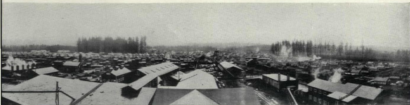
City of Onalaska, Washington. J. W. Luke, Portland, Oregon; Consulting Engineer
