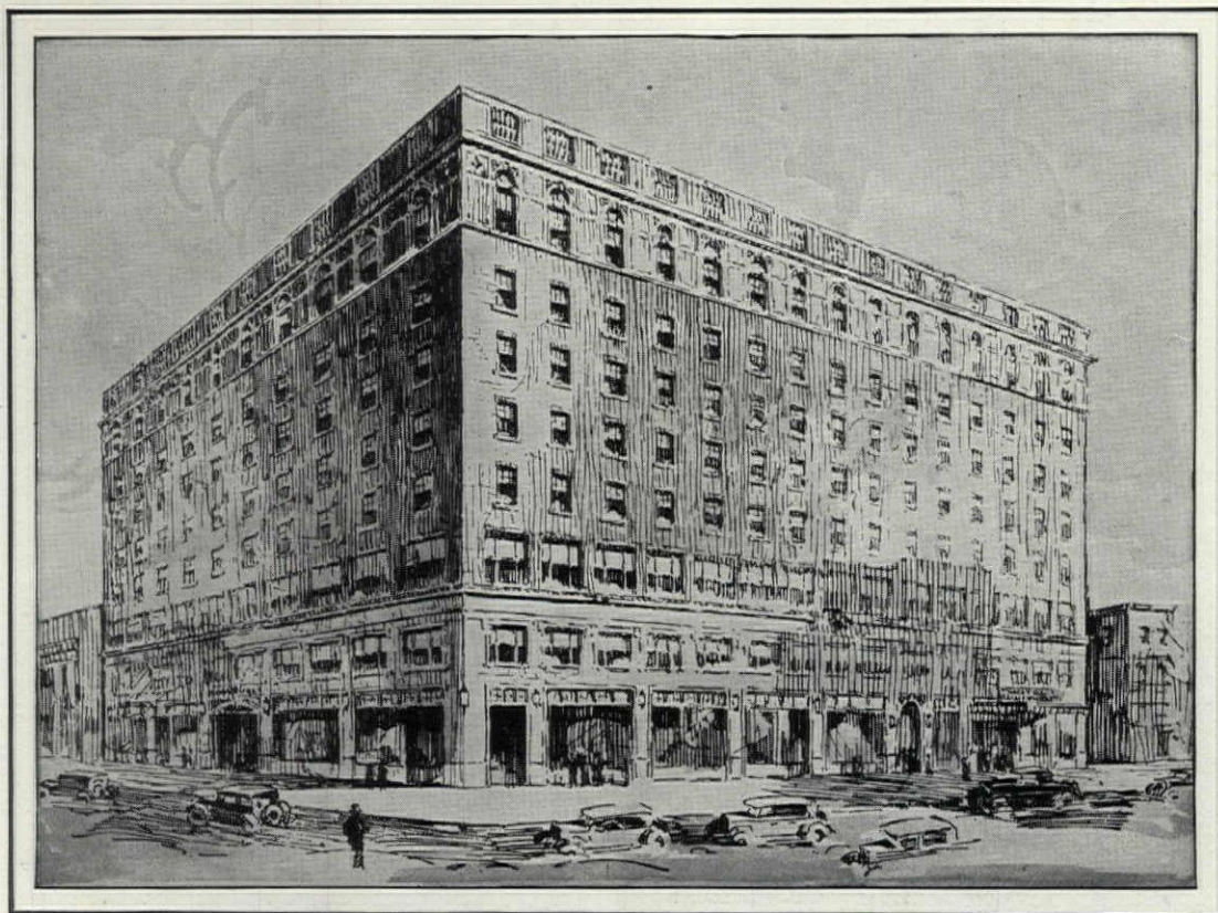
The Roosevelt Hotel, St. Louis, Missouri, a magnificent new hostelry, given the permanent protection of a Carey Built-up Roof. Widmer Engineering Company, Architects and Engineers, St. Louis, Missouri.
