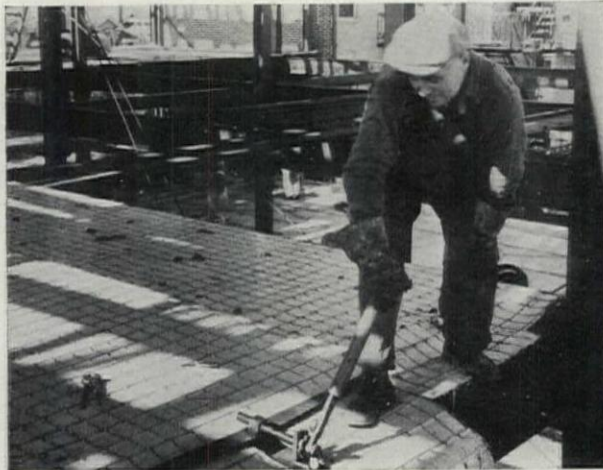
Stretching Welded Mesh Reinforcing Fabric
