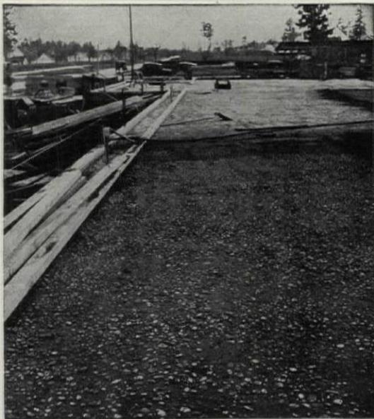
A Con-Tex Bond Surface on the top surfaces of underslabs enables a perfect topping to be applied as a finishing operation
