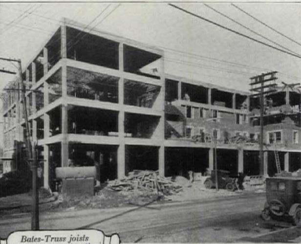
*Bates-Truss joists in concrete construction St. Louis Mo.*
