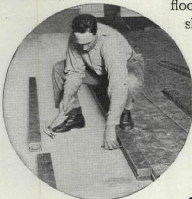
Lasting smoothness — durability — resiliency — these three essential qualities are combined to a greater degree in BLOXONEND than in any other flooring material. Laid directly over concrete without embedded sleepers.
