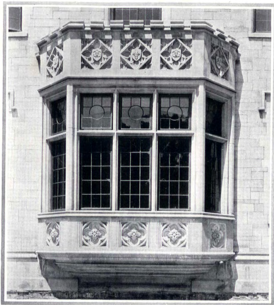
Detail, Oriole Bay Window, Dormitory, Marygrove College, Detroit, Michigan. D. A. Bohlen & Sons, Architects. Rough sawed VARIEGATED Indiana Limestone Random Ashlar with buff trim
