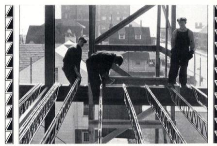
Workmen are here shown installing Havemeyer Trusses on the Biarritz Apartments, Atlantic City. After the trusses are spaced, they are firmly bridged and covered with reinforcing fabric or metal lath, ever which the concrete slab is poured without requiring formwork.
