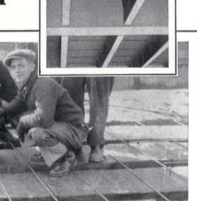
Note the rigidity of Meyer Steelforms. The heavy 16-gauge sheet steel permits walking and trucking over the forms without bending them. This speeds up work on the job.
