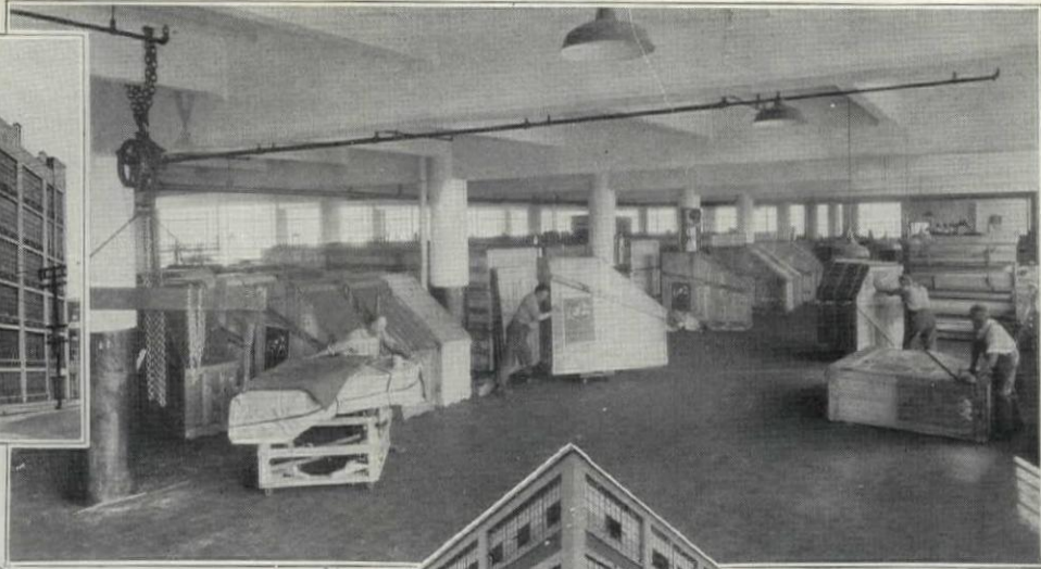
Above— Shipping room, Steck Piano Co., Boston. Only one man necessary to move these crated pianos. Note size of casters. This demonstrates the smoothness of Bloxonend.
