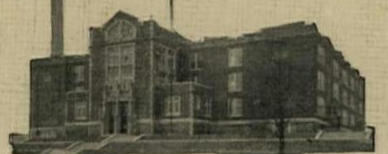
Public School No. 15, Paterson, N. J. Lee and Hewitt, engineers and architects, New York, N. Y.
