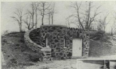
A typical installation in a suburban community.
