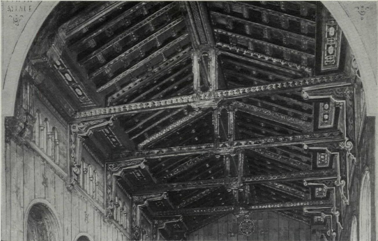
Main Roof Trusses as They Will Appear When Finished
