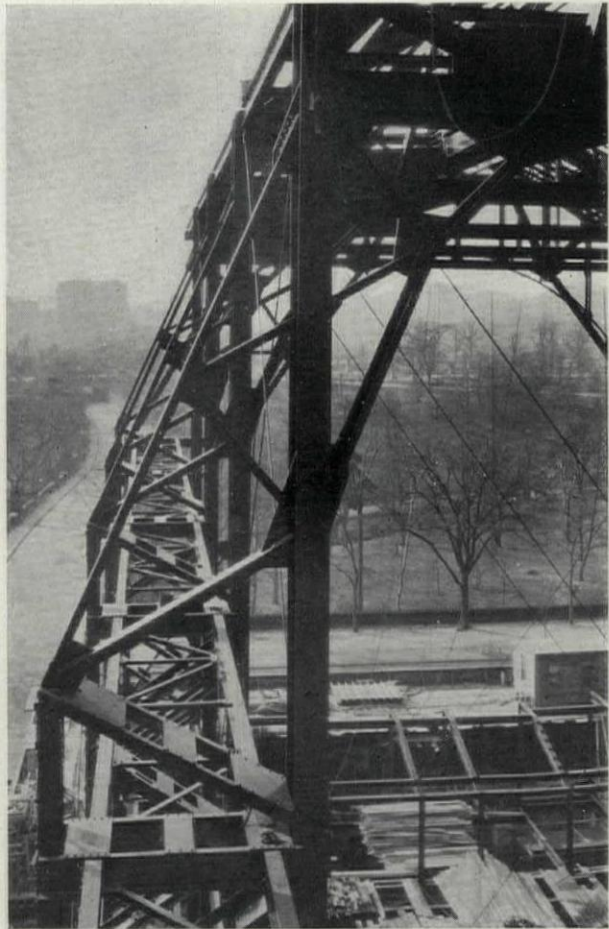
Supports and Bracing
