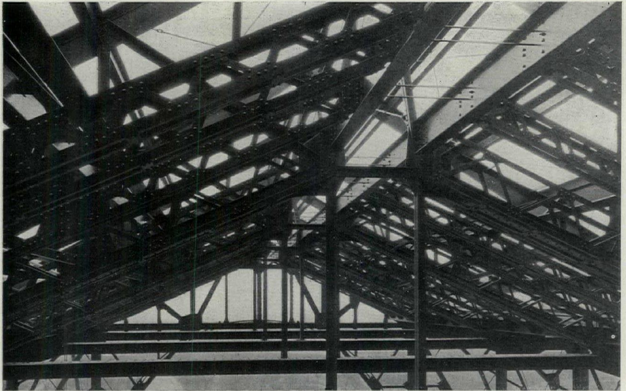
The Main Roof Trusses
