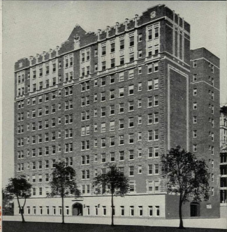
Apartment Hotel, 180 E. Delaware Place, Chicago Architect and Engineer: B. Leo Steif & Co. Heating Contractor: Schampel & Dougherty
