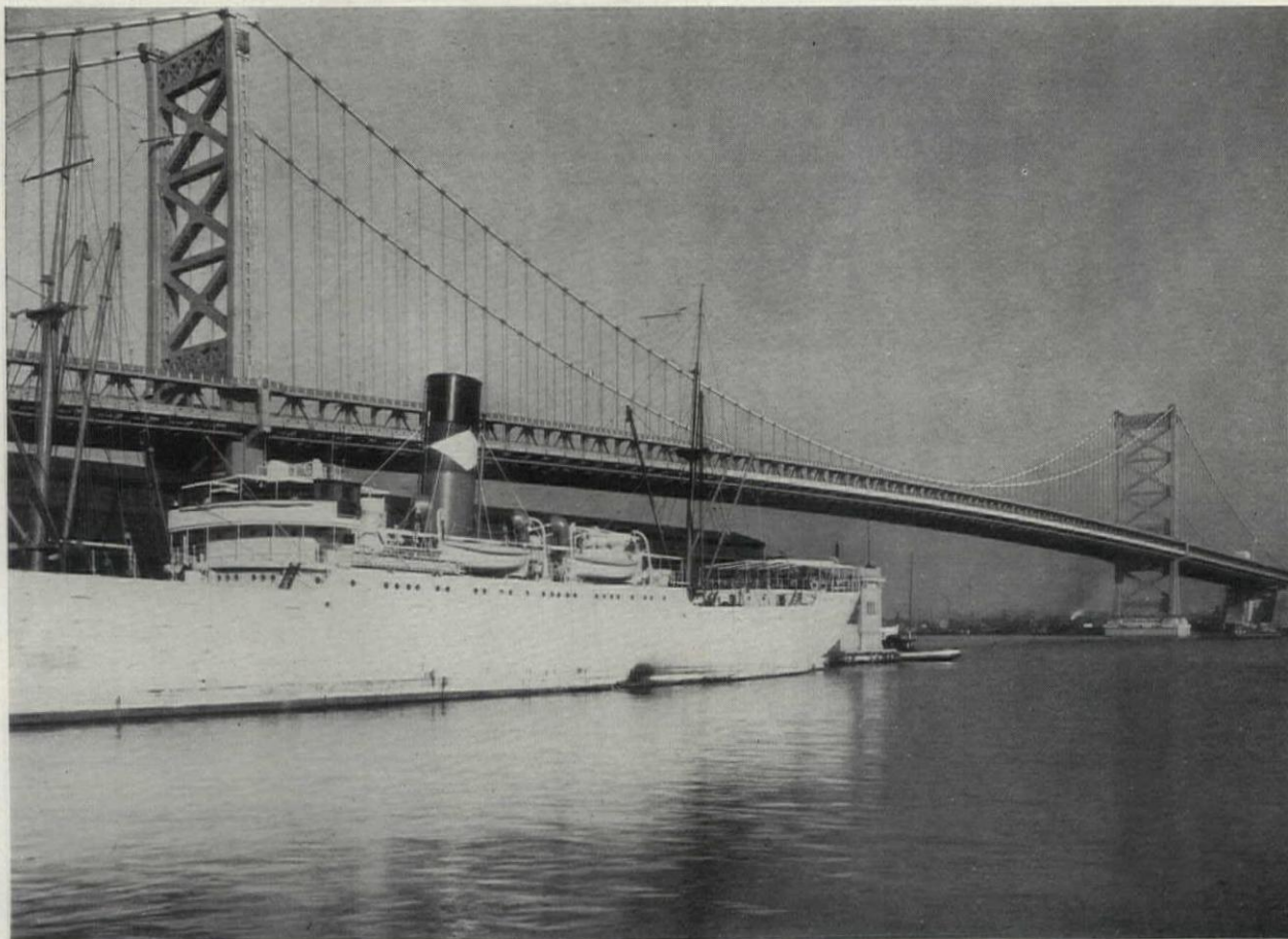
General View of the Bridge from the Water Front
