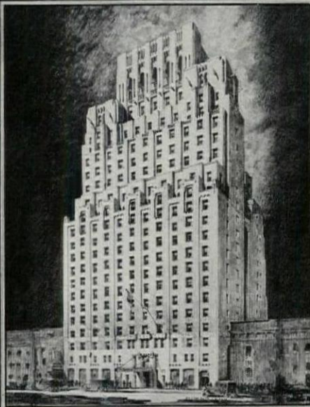
Signal Engineering Fire Alarm System installed in Piccadilly Hotel, New York City. Architects, George & Edward Blum and S. Walter Katz. Consulting Engineer, Charles Mayer. Electrical Contractor, Thor Electric Co., Inc.
