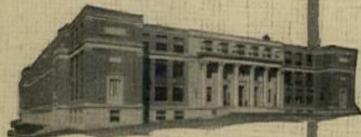
Worcester Junior High School, Worcester, Mass. J. D. Leland & Co., architects and engineers, Boston, Mass.
