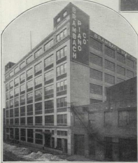
Brambach Piano Co., New York City. Plant floored throughout with Bloxonend.
