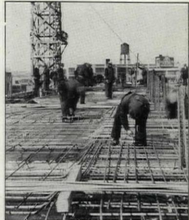
The photographs shown here were taken during the installation of Havemeyer Bars in the Mail Order Building of Sears, Roebuck & Co., Boston. George C. Nimmons, Architect; Hegeman & Harris Co., Contractors
