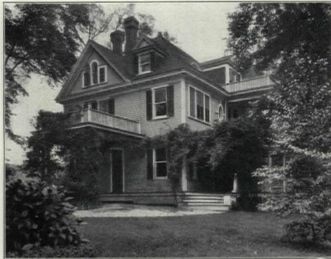
The first domestic Petro was installed in this home of Cyrus Field Judson, November, 1923. This original burner is giving most satisfactory service.
