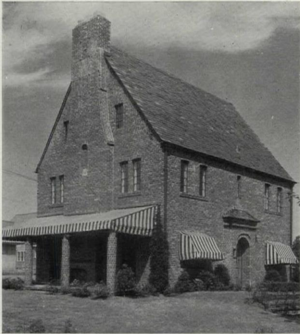
Fig. 7. Variety in Brick Texture John T. Briggs, Architect
