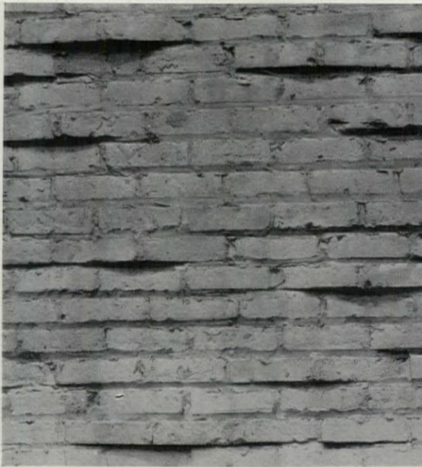
Fig. 10. Detail of Brickwork Shown in Fig. 11 Russell Walcott, Architect
