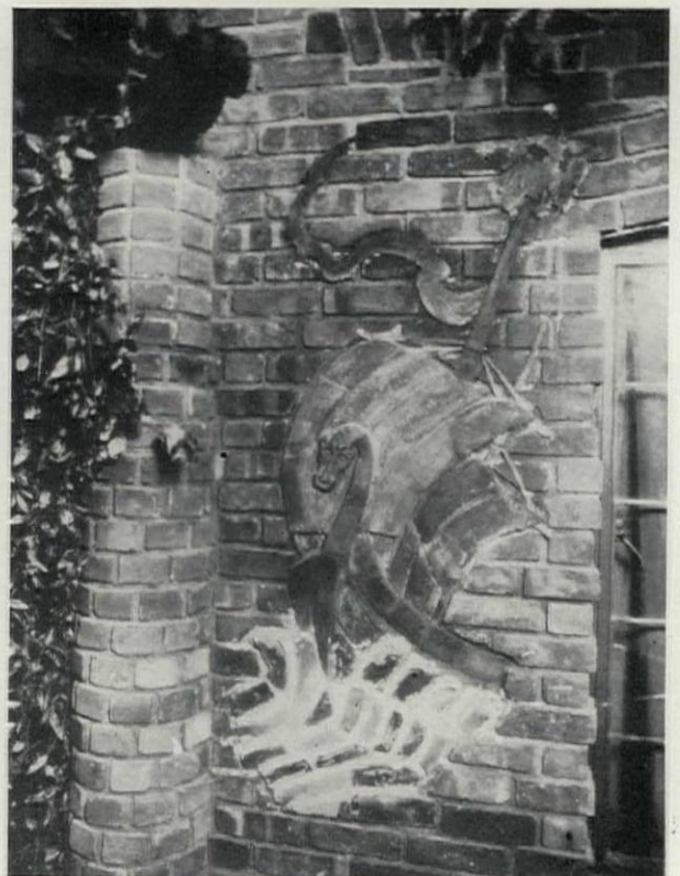
Fig. 13. Ship Design, Simply Executed John T. Briggs, Architect
