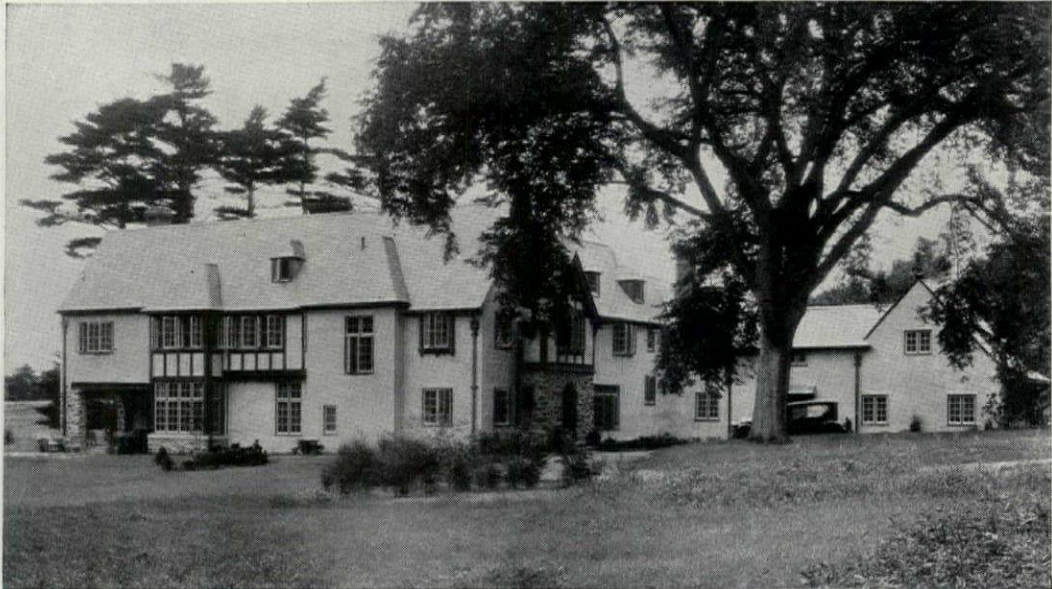
Know Electrol by the Homes It Heats
