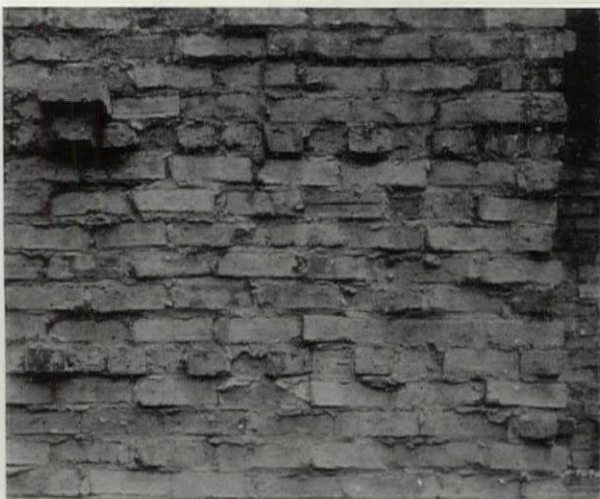
Fig. 9. Detail of Brickwork Shown in Fig. 8
