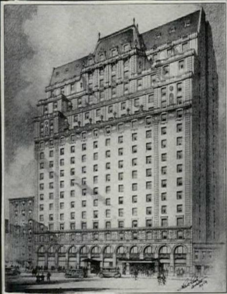
Signal Engineering Fire Alarm System Installed in Paramount Hotel, New York City
