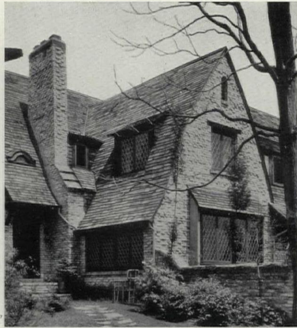
Fig. 8. Skintled Brickwork S. S. Beman, Architect
