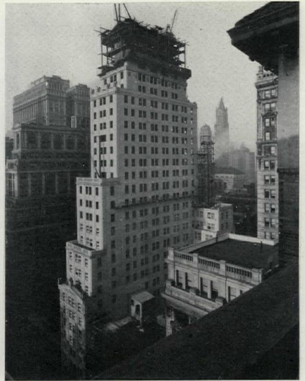
Building for National City Company, New York McKim, Mead & White, Architects Built on Cost Plus Percentage Basis George A. Fuller Co., Builders
