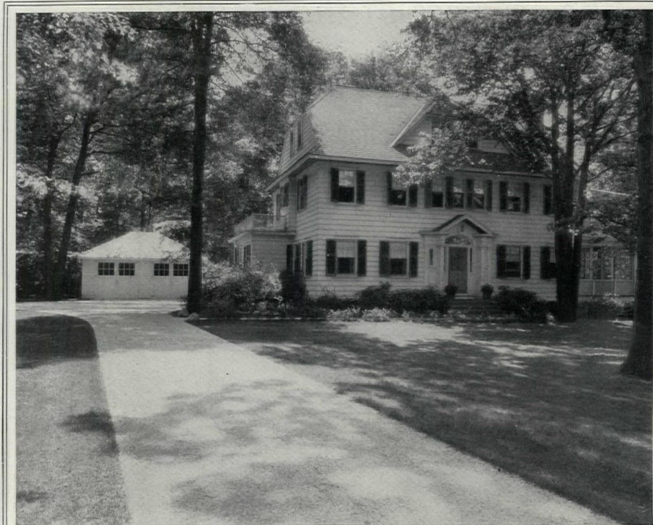
Roadway and Sidewalk—Residence of Nathan C. Johnson, Consulting Engineer, Englewood, New Jersey. James L. Bried, Contractor, Englewood, New Jersey.
