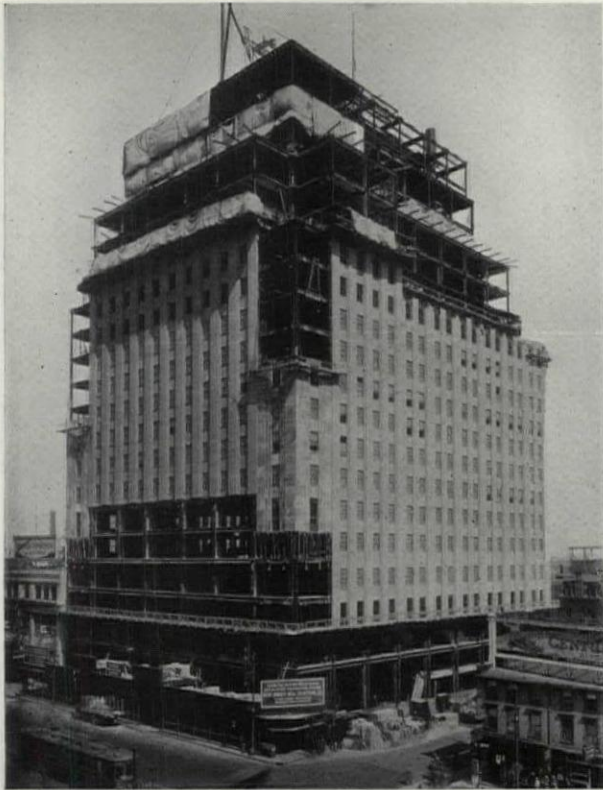
New Jersey Bell Telephone Building, Newark
