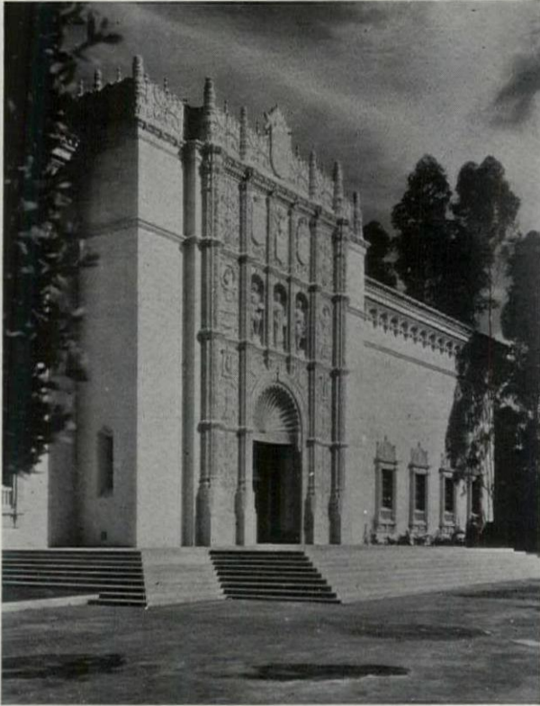
Intricate Design in Cast Stone, Fine Arts Building, San Diego Templeton, Johnson & Snyder, Architects
