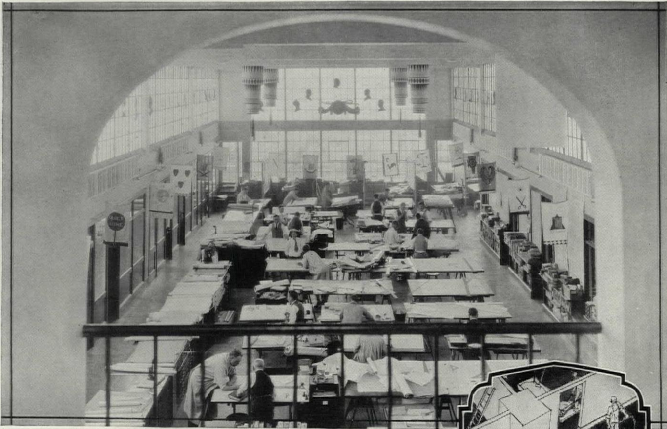
Battleship Gray Colormix Floor in drafting room of Walker & Weeks' office, Cleveland, Ohio. Approximately half their floor area is of exposed cement finish all permanently colored and hardened with Colormix and Dycrome. Walker & Weeks, Architects.
