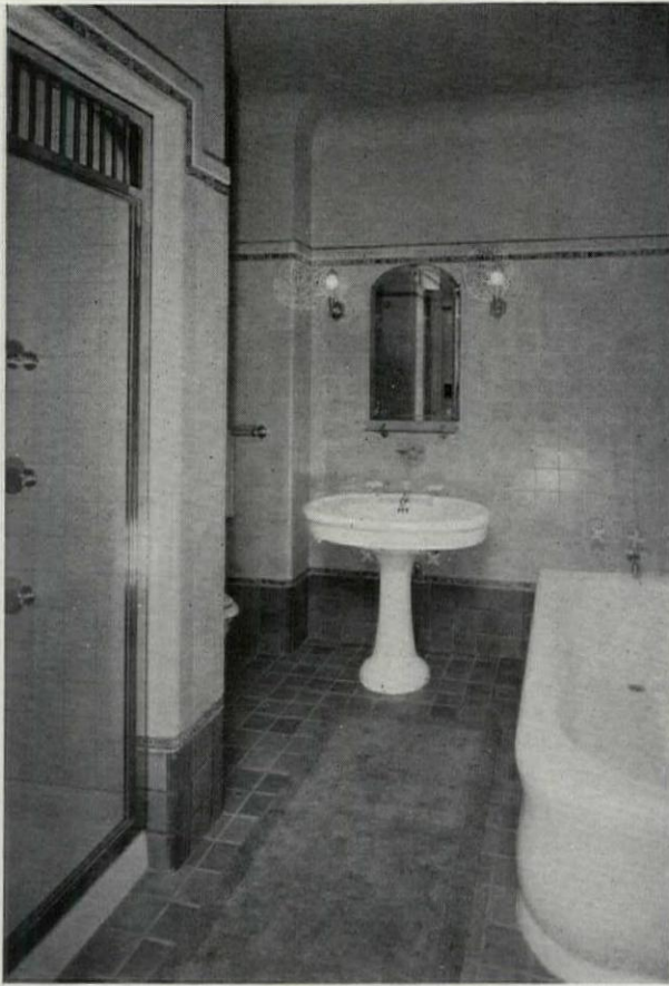
Built-in Tiled Shower with Ventilating Plate Glass Door
