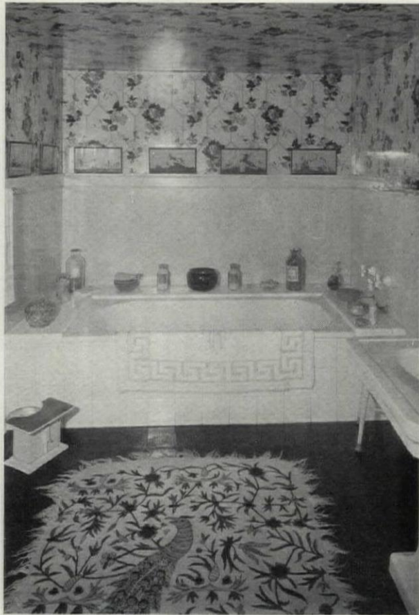
Convenient Tile Shelf Built Around the Tub
