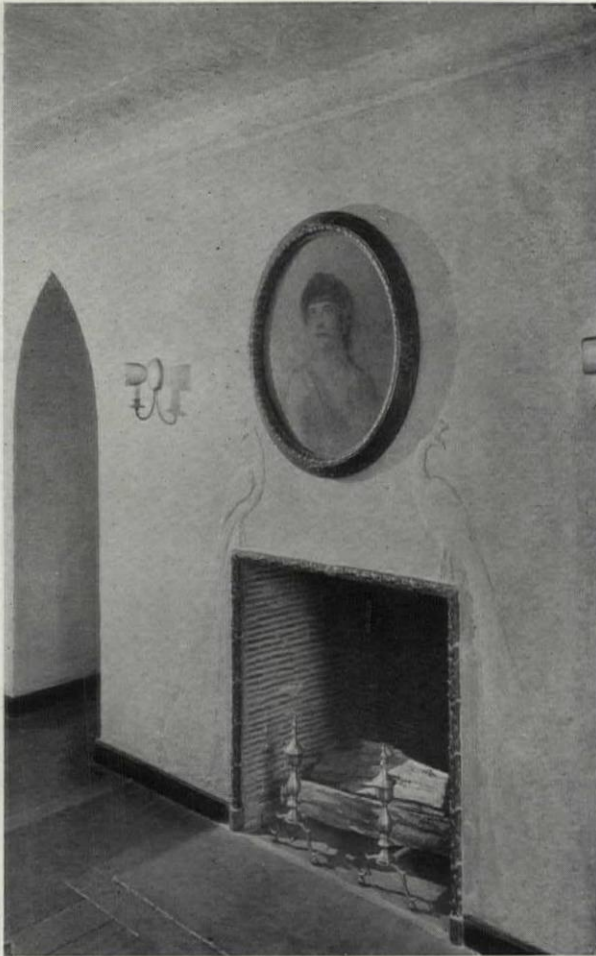
Palm-finished plaster is here used appropriately. The peacocks worked in flat relief were designed to help frame the portrait above the fireplace
