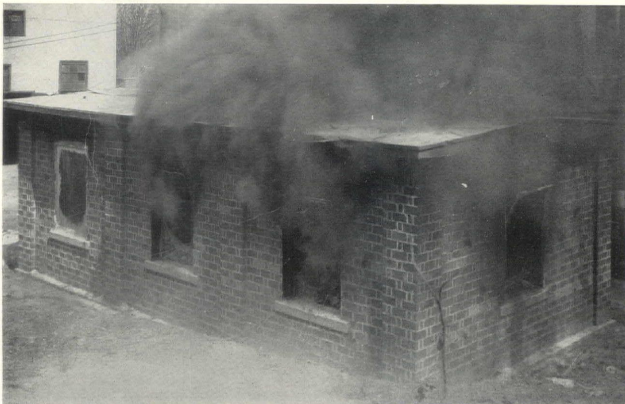
View During a Fire Intensity Duration Test of Small House Shown Opposite
