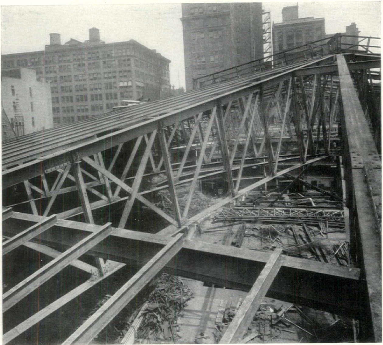
Long Roof Trusses of Madison Square Garden in Perfect Condition after 35 Years of Service
