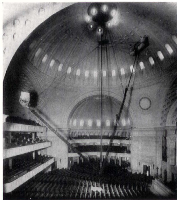
Booms Used in Refinishing Interior
