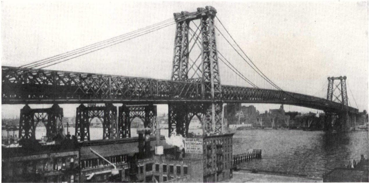
Williamsburg Bridge, New York. Central Span Only Supported by Cables
