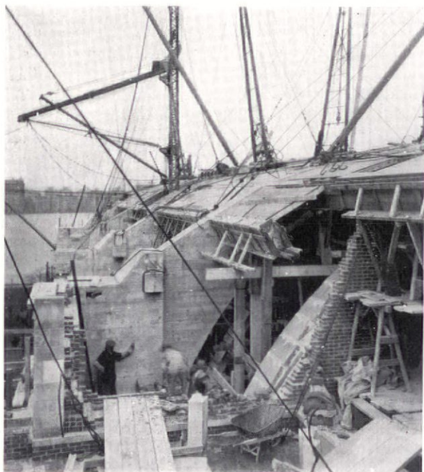
Tops of Ribs, Roof Slabs and Beams, Church of the Heavenly Rest
