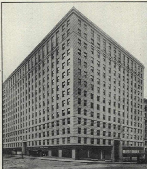
NATIONAL PRESS BUILDING, WASHINGTON, D. C. TONTINE-EQUIPPED
