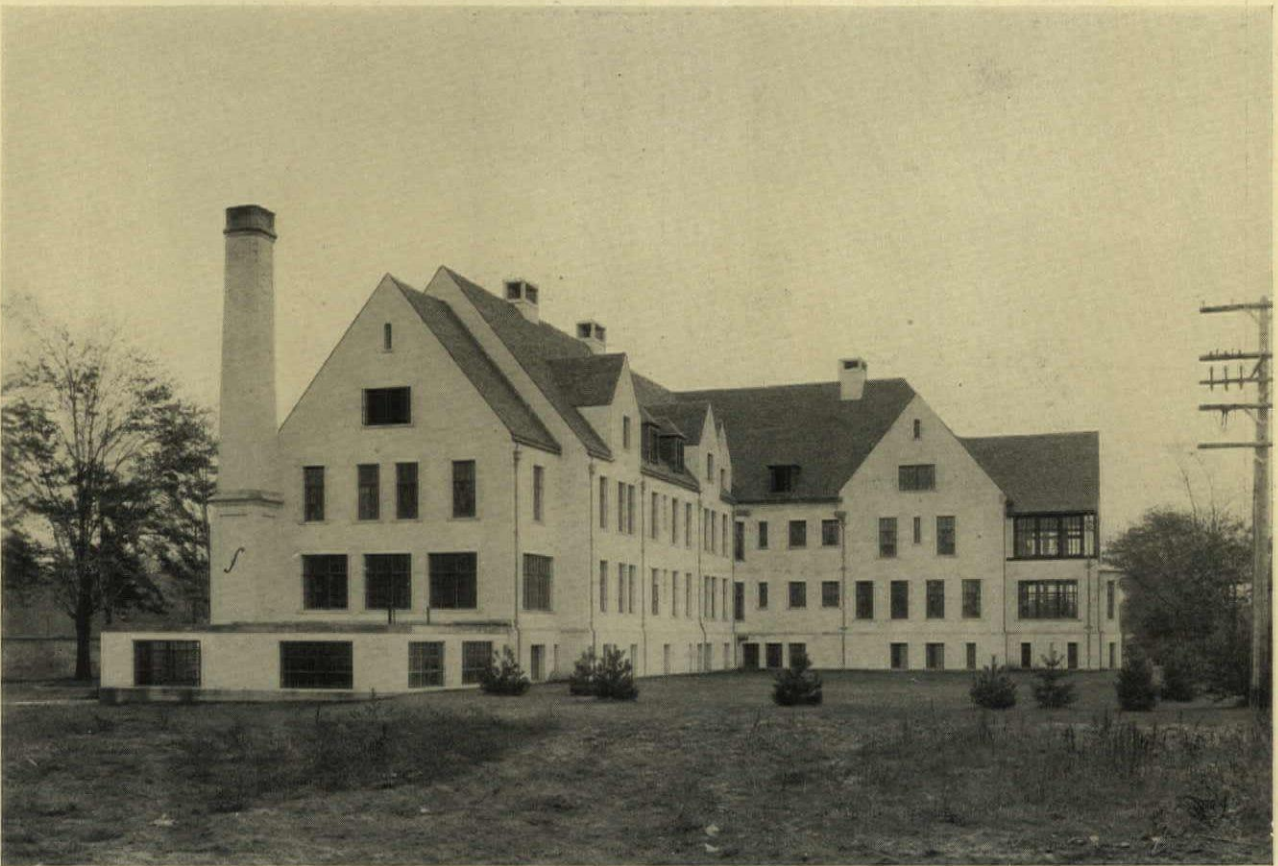
END AND REAR ELEVATIONS COTTAGE HOSPITAL, GROSSE POINTE, MICH. STEVENS & LEE, ARCHITECTS
