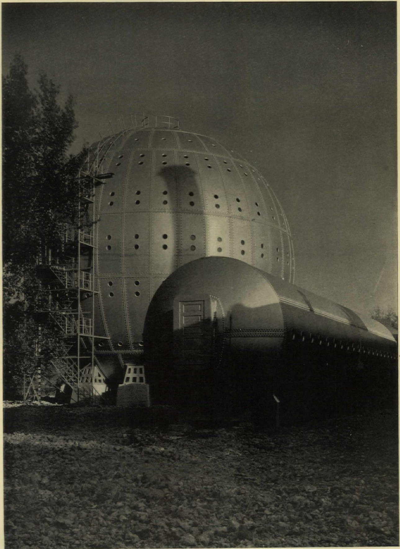
AIR PRESSURE WARD, CUNNINGHAM SANATORIUM, CLEVELAND
