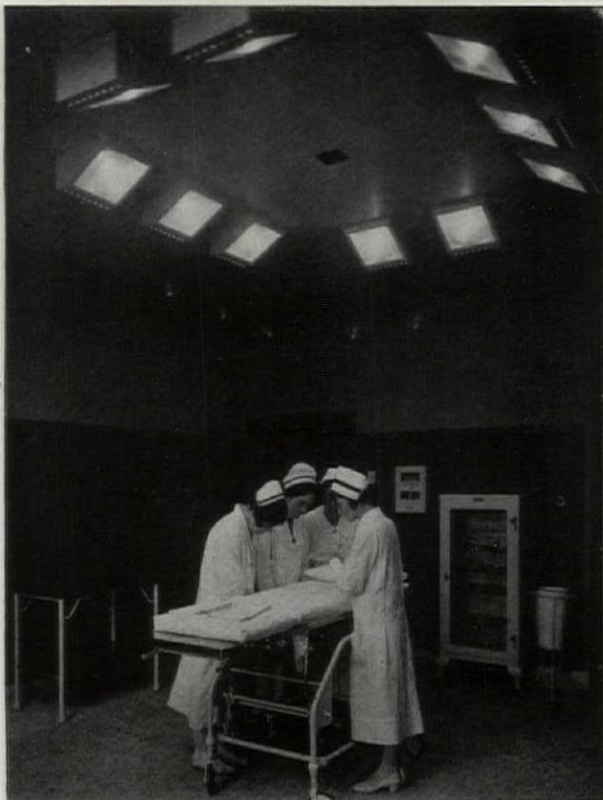
Floodlights of a Focusing Type Leave the Table Free from Shadows
