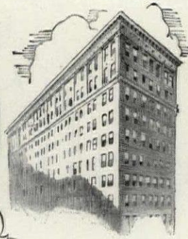
This Office Building at 90 Worth St. is one of many of New York's famous Skyline Te-pe-co equipped.
