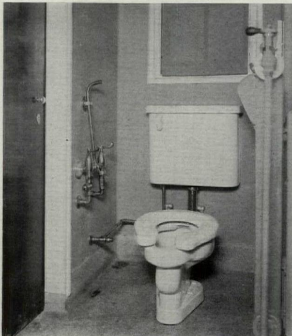
Fig. 15—Detail of Private Room Toilet, Showing Bed Pan Washing Device
