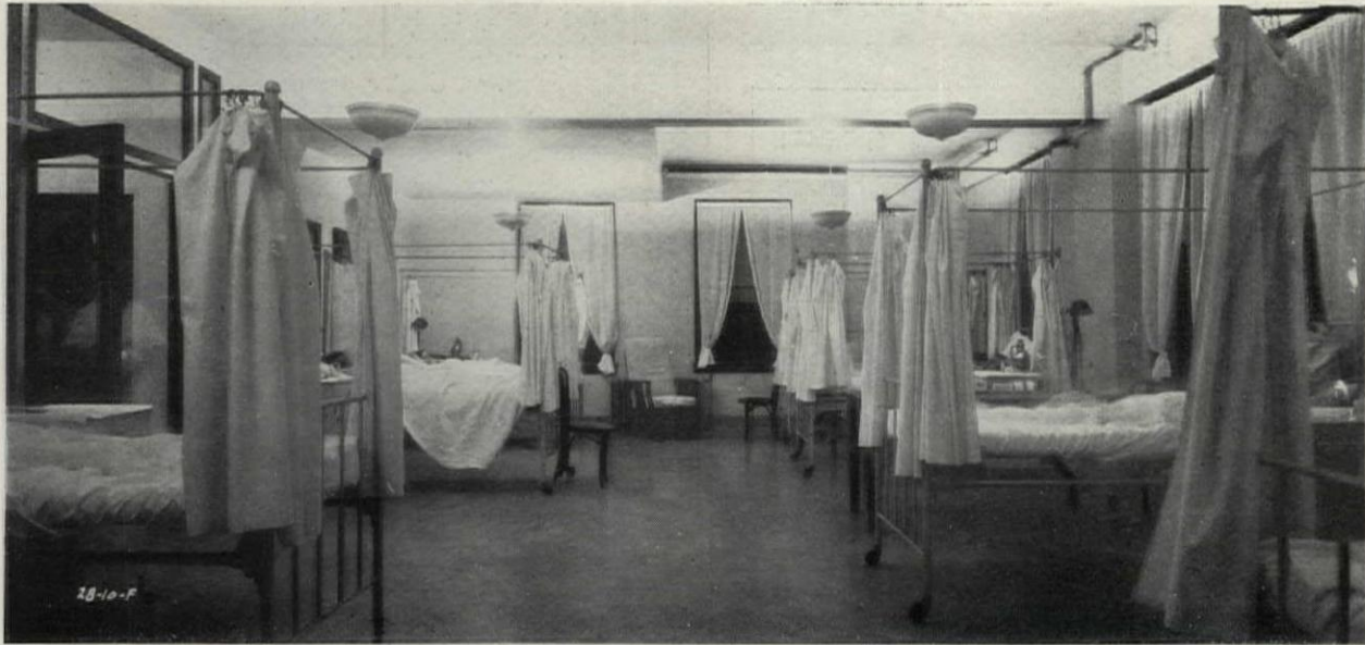
Diffused Light is Supplied in the Ward by Indirect Fixtures
