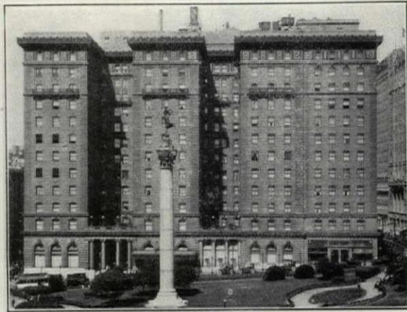
St. Francis Hotel, San Francisco,—comfortably, economically heated with Johnson Oil Burners—also uses Johnson oil burning equipment in its kitchen. Where comfort and efficiency is paramount you find Johnson installations.
