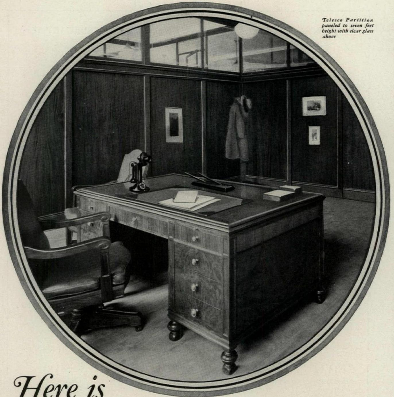
*Telesco Partition paneled to seven feet height with clear glass above*
