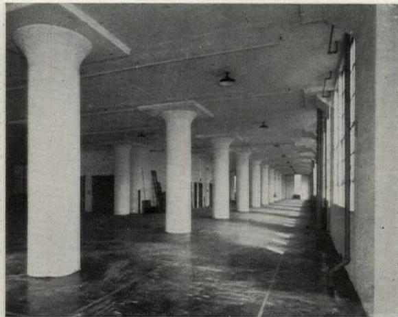
Typical Reinforced Concrete Girderless Floor Construction with Drops Over Columns and Half Drops at Walls. Cass Gilbert, Architect
