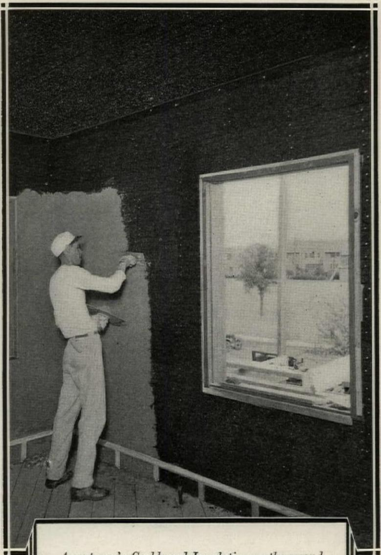
*Armstrong's Corkboard Insulation on the second floor of Mr. H. B. Thompson's residence at Dallas, Texas. The plaster is being applied directly on the cork, without lath.*
