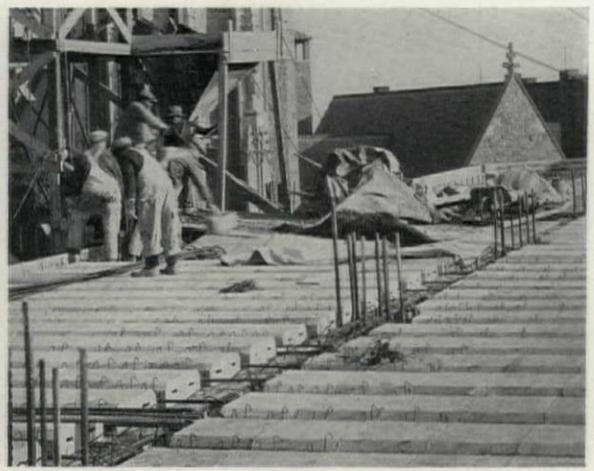
Concrete Rib Construction with Gypsum Block Used As Fillers on a Building in Baltimore
