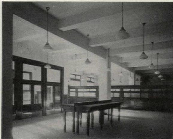
Typical Reinforced Concrete Beam-and-slab Construction as Designed for a New York Post Office. A. S. Alschuler, Architect
