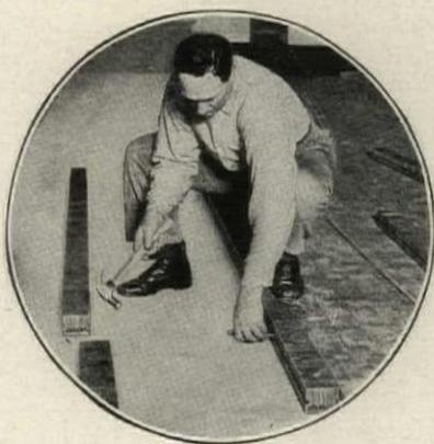
By our lateral nailing method, Bloxonend is laid directly over wood-floated concrete slab, eliminating sleepers and fill and effecting a saving in ceiling height.
