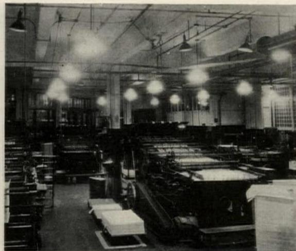
Color printing. Press room. General illumination. 300-watt clear lamps, diffuser. Spacing 12 x 12'. Lamps 12' above floor. Ceiling 14'. Illumination level 18 foot-candles. Projector type equipment with 200-watt daylight lamps. Color identification unit at inspection table. Waverly Press, Baltimore
