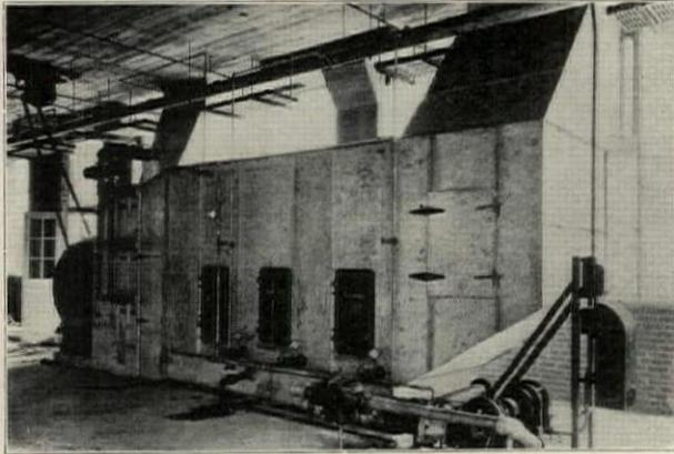
A Webster type B dehumidifier in service at the Brandle and Smith Candy Factory, Philadelphia. This installation as well as the distributing ducts are made of rust-resisting ARMCO Ingot Iron. The continual exposure to moisture laden with carbon dioxide necessitated the dependable protection of pure iron.
