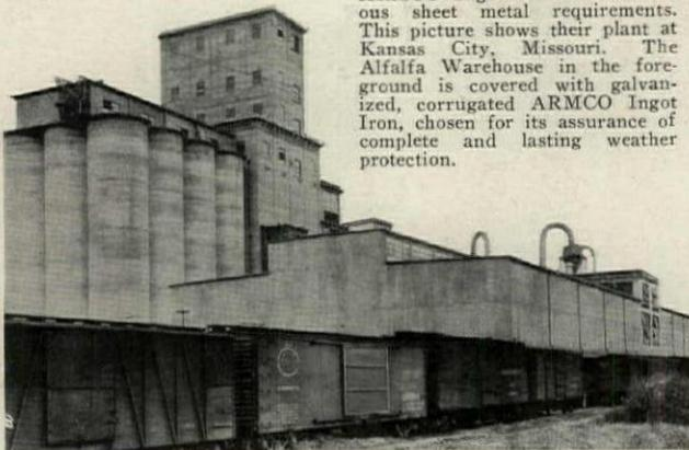
The Purina Mills is one of the many great industries that use ARMCO Ingot Iron for numerous sheet metal requirements. This picture shows their plant at Kansas City, Missouri. The Alfalfa Warehouse in the foreground is covered with galvanized, corrugated ARMCO Ingot Iron, chosen for its assurance of complete and lasting weather protection.
