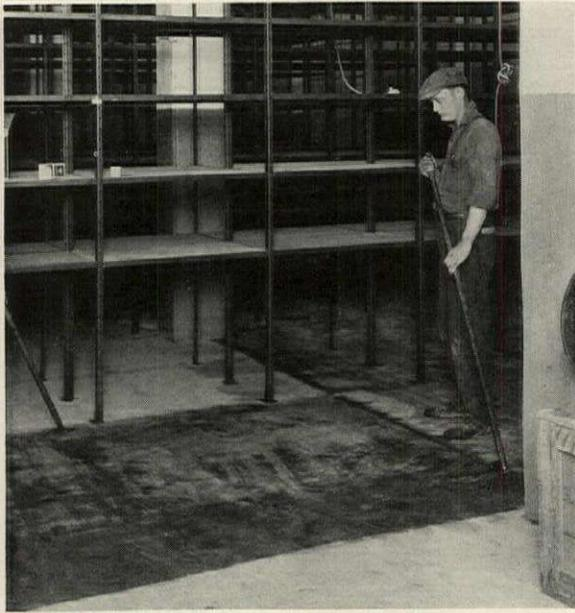
Applying a Coating to a Concrete Floor to Make it Hard and Dustless
