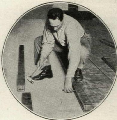
*Bloxonend lays rapidly and can be installed in old plants with but slight interference to daily operations.*
