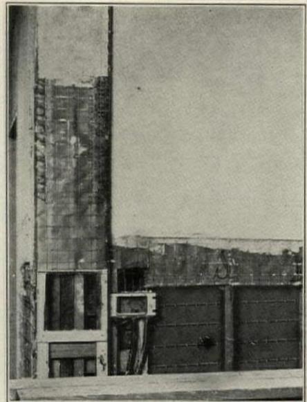
**REQUIRES NO NEW APPLICATION METHODS—** Plaster goes up easily on RIBBED STEELTEX with long, smooth sweeps of the trowel. The level, rigid sheets save mud on the scratch coat and assure even thickness of plaster slab with uniform reinforcement. Note fibrous, absorptive backing, furred-out steel reinforcing fabric, and new V-rib stiffeners on back of sheet.
