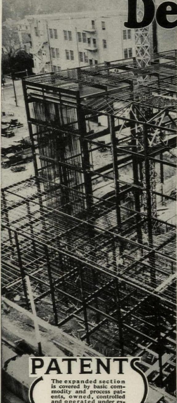
NO WELDS IN STRESS—one piece of steel—expanded—without rivets, bolts or welds in shear or tension—these are the features responsible for the rapid gain in Bates-Truss Joist popularity.
