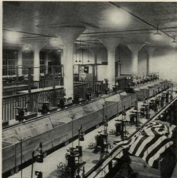
Flag manufacturing. General lighting 500-watt white bowl lamps, dome reflector. Outlets 20 x 20'. Lamps 13' 6" above floor. Ceiling 14'. Ceiling, walls white; illumination level 10 foot-candles. Local lighting 15-watt lamps. Annin & Company, Verona, N. J.
