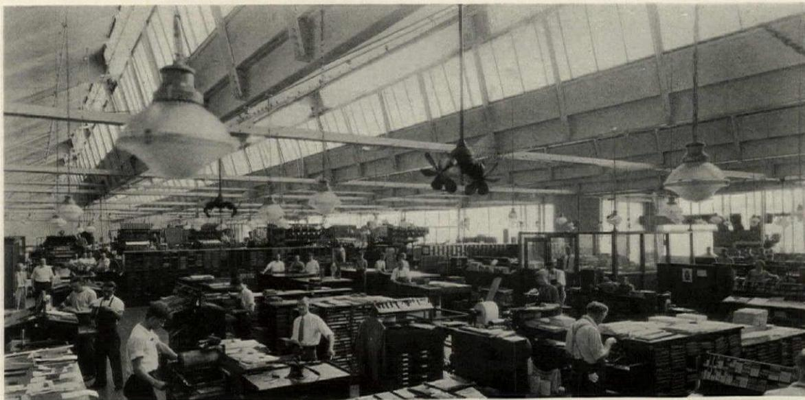
Interior of Modern Printing Plant for Mack Printing Company. Shown at the Top of Page. Sawtooth Construction with Maximum Daylight Illumination and Super-span Truss Construction, Eliminating all Columns
