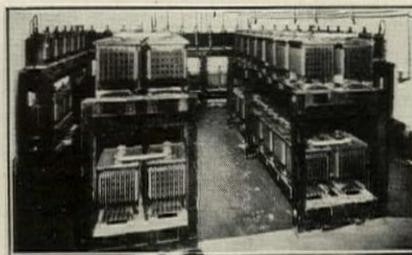
THIS DEPENDABLE EXIDE protects lights in Baldwin administration building. The 25-cell Exide, Chloride type, in background, supplies current for entire telephone system throughout plant.
