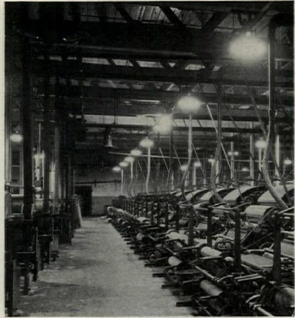
Textile mill. Rough fiber carding. 200-watt white bowl lamps, dome reflectors. Outlets 16 x 15'. Lamps 14' above floor. Roof trusses 16'. Ceiling white, side walls white and glass. Illumination level 10 foot-candles.
