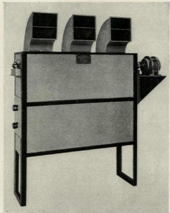
A Unit Heater Designed for Floor Mounting
