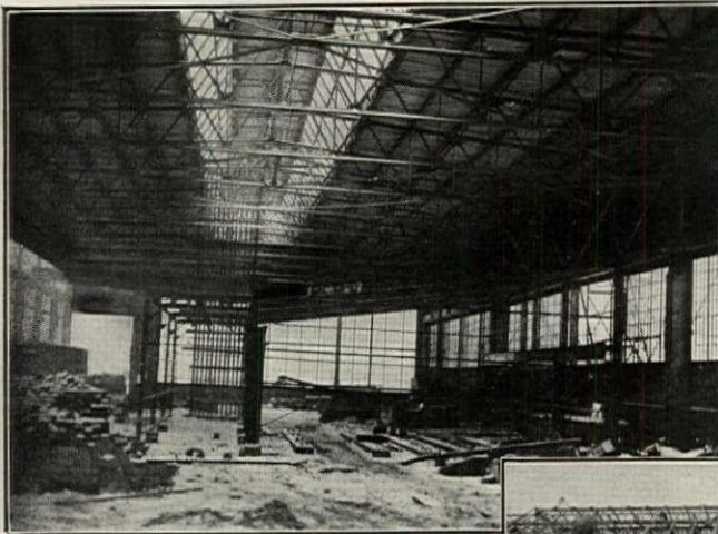
Interior of Bliss & Laughlin plant showing clear light reflecting under surface of Gypsteel roof deck.
