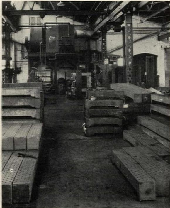
Metallic Hardcured Concrete Floor for Heavy Duty
