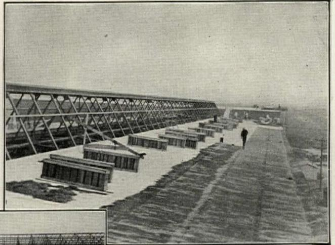
Gypsteel roof being laid in severe weather last January.
