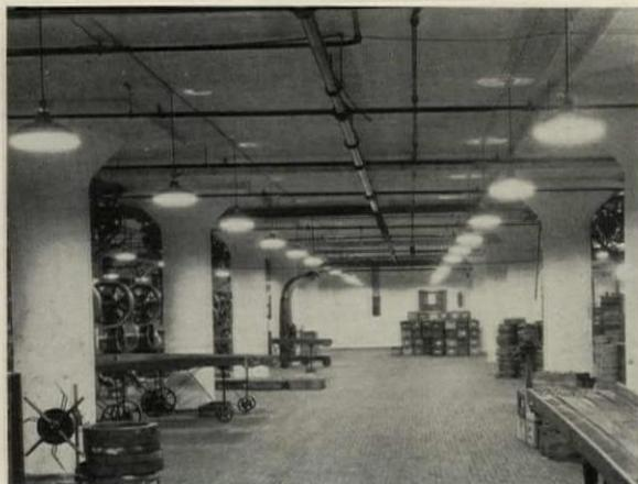
Hardware manufacturing. Blanking punch presses. 150-watt white bowl lamp, dome reflector. Outlets 10 x 10'. Lamps 8' 6" above floor. Ceiling 10'. Walls and ceiling white. Illumination level 12 foot-candles.
