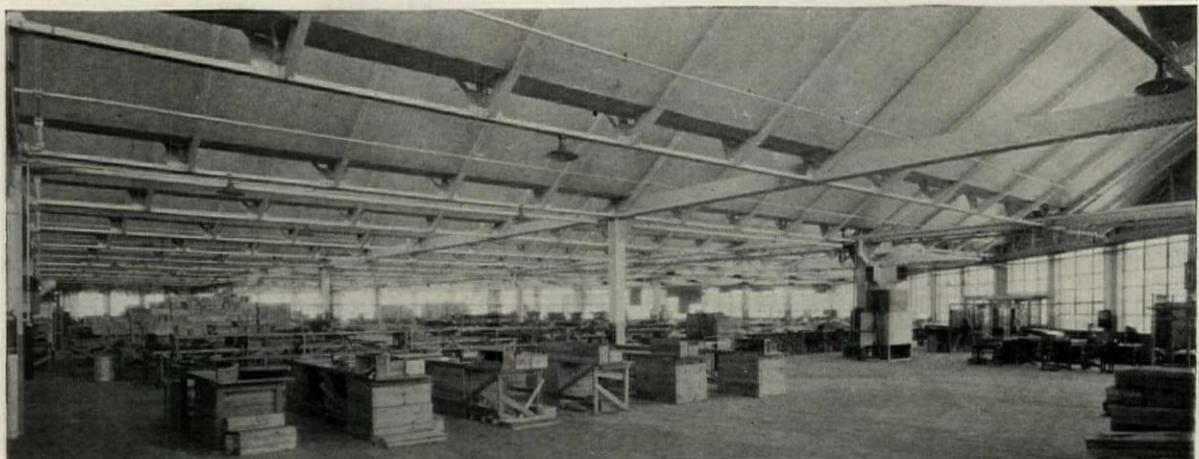
Interior of Modern Radio Manufactory of Atwater Kent Manufacturing Company, Using Super-span Sawtooth Skylight Showing Reflecting Value of Light Colored Roofing Material on Slope of Adjoining Sawtooth
