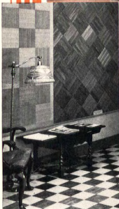
A corner of the exhibit, showing *CELLized wood blocks for walls as well as floors. Panel at left, white and red oak, laid alternately; at right, red gum, maple and walnut blocks.
