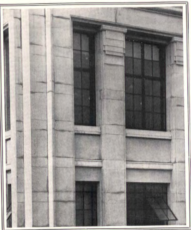
The illustration at the left is a typical example of weeping joints. Notice the ugly stains.
