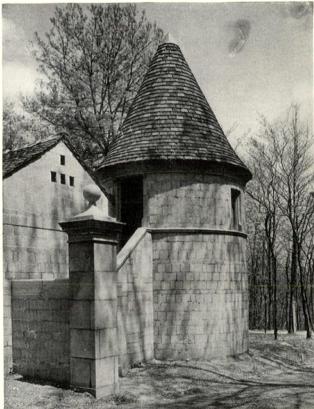
● A charming time-worn texture was given the walls of this and other buildings on the place of Michael Gavin, Jericho, L. I., by using cinder blocks of varying size which had been sprayed with water while still soft. These walls called for a roof that also simulated age, so Hopkins and Dentz, the architects, chose IMPERIAL Shingle Tiles. In color and texture they are amazingly faithful reproductions of tiles which have seen centuries of use.
