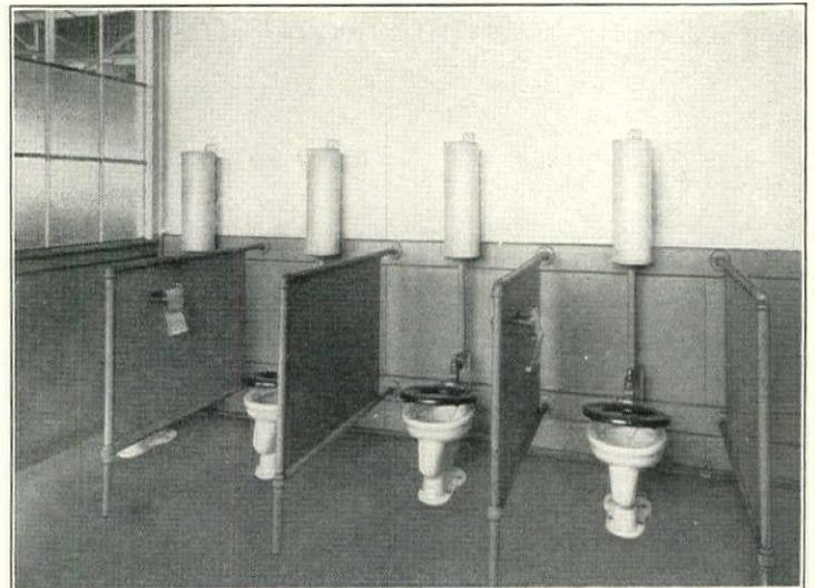
*A typical installation of Vogel Number Ten Closets. Photograph taken in the Pusey & Jones plant, at Wilmington, Del. A closet similar to these on an endurance test has flushed 230,000 times without even a washer being renewed.*
