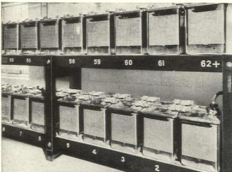
HERE IS AUTOMATIC PROTECTION FOR LIGHTS AND POWER. Picture shows a typical Exide Emergency Lighting Battery in glass jars, which make inspection easy. The cells are arranged on neat, compact racks and can be placed in the basement of buildings or any other suitable location. They take up little space and the arrangement is flexible.
