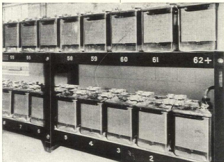
*AUTOMATIC PROTECTION for light and power. Picture shows typical Exide Emergency Lighting Battery in glass jars, which make inspection easy. Cells are arranged in neat, compact racks, and are placed in basements of buildings near the engine room. They take up little space and the arrangement is flexible.*
