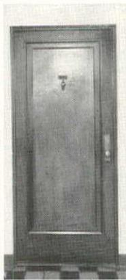
“... it is unique in this result. The Frame closely engages the tile—The wall anchors are positive in their function—The plaster is bonded and reinforced over the sides of the Frame
