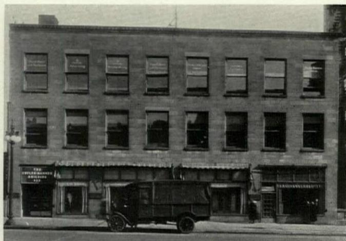
The building before remodeling. Notice how the new facade above has been based upon the fenestration in this before picture. The spandrel areas between upper and lower window has been designed to give a feeling of height and dignity to the windows. The old-fashioned transoms over the display windows are omitted in the new design.
