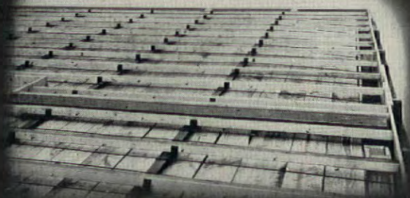
(3) The finished concrete form with wooden sleepers and \frac{1}{4} " steel reinforcing rods in place.
