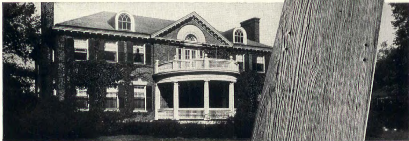
Home of Mr. N. W. Willard, Asst. to the President of the Atchison, Topeka and Santa Fe Railway, Riverside, Ill. Roofed with 35 squares of 8" x 16" Quarry Blue Eternit TimberTEX Asbestos-Cement Shingles.
