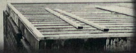
(4) The steel and concrete floor complete. Finished flooring will be nailed to the sleepers.
