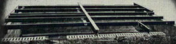
(1) This picture shows the entire layout of steel in position on foundation walls.
