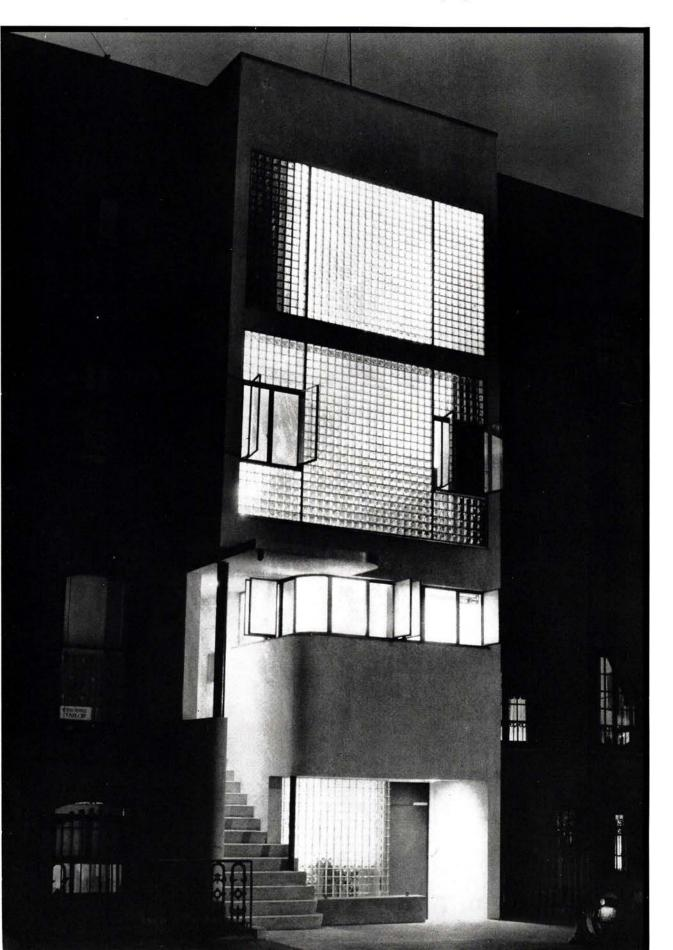
Legal, engineering, and human requirements nicely balanced and fulfilled. The glass wall of the air conditioned living room on the top floor admits sunlight and obscures an unattractive prospect. The guest room because it is used only occasionally has no air conditioning, hence windows.
