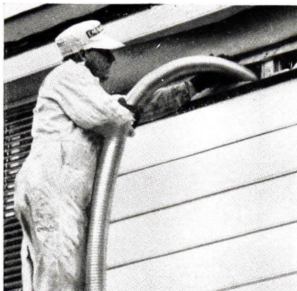
• No building alterations are necessary when Eagle Home Insulation is installed. To gain access to hollow spaces between wall studs, operator removes a few pieces of siding, or a few bricks, or makes small openings in stucco.
