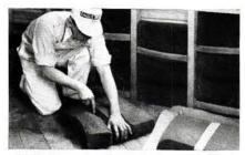
· Eagle Home Insulation is also available in "bat" form for new construction. These bats, or pillows, are 15" by 18" and 35%" thick. Easy to fit between wall studdings and attic joists.
