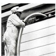
· No building alterations are necessary when Eagle Home Insulation is installed. To gain access to hollow spaces between wall studdings, operator removes a few pieces of siding, or a few bricks, or makes small openings in stucco.
