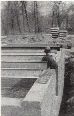
ft. foundation walls waterproofed with emulsified asphalt. ght, The I-beams in place for floor construction.
