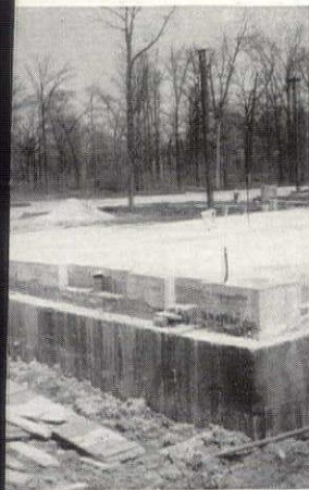
ft. foundation walls waterproofed with emulsified asphalt. ght, The I-beams in place for floor construction.
