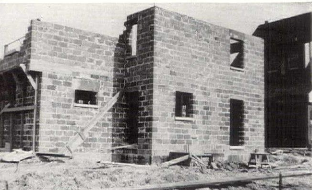
Wall of Haydite building units in course of construction, stucco applied directly to exterior walls, metal lath and plaster to inside walls.
