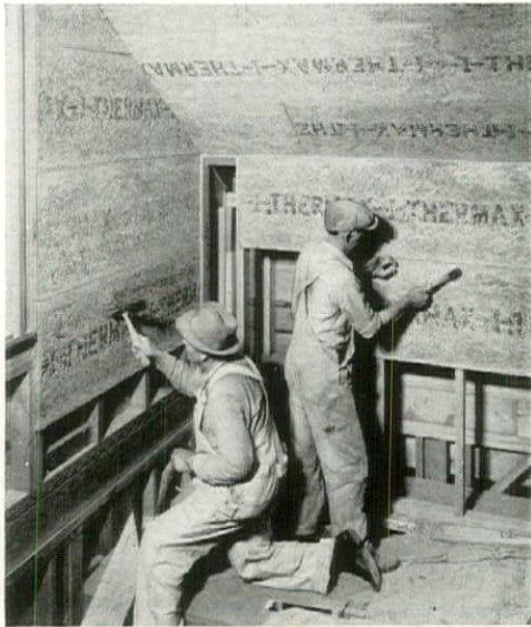
INSULATING BOARD ON WOOD FRAME
