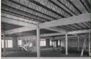
TRUSCON OPEN TRUSS STEEL JOISTS PROTECT THE THREE FLOORS AND ROOF OF THE HORTICULTURAL BUILDING, GREAT LAKES EXPOSITION, CLEVELAND, OHIO
