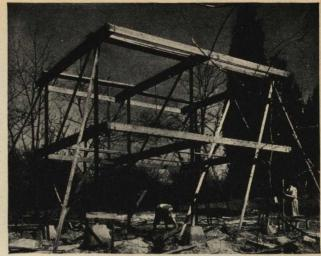
LALLY COLUMNS AND BUILT-UP AND NOTCHED BEAMS
