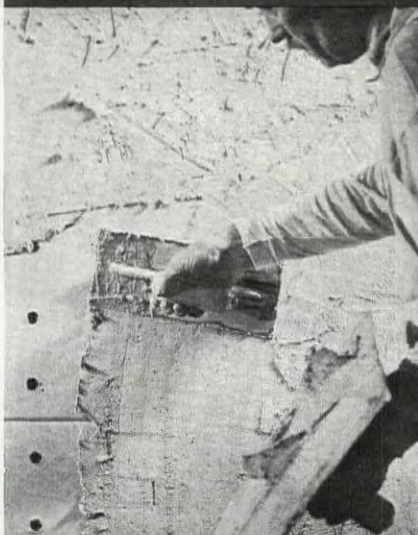
Red Top Plaster being applied to Perforated Rocklath.
