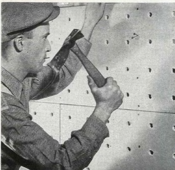
Perforated Rocklath being applied to studs — goes up quickly, easily.
