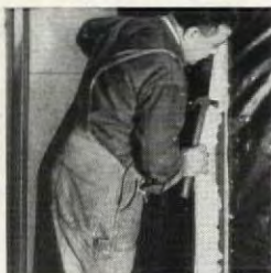
Showing stud application. Backed with heavy water-proof paper. RED TOP STRIP WOOL is easy to nail.
