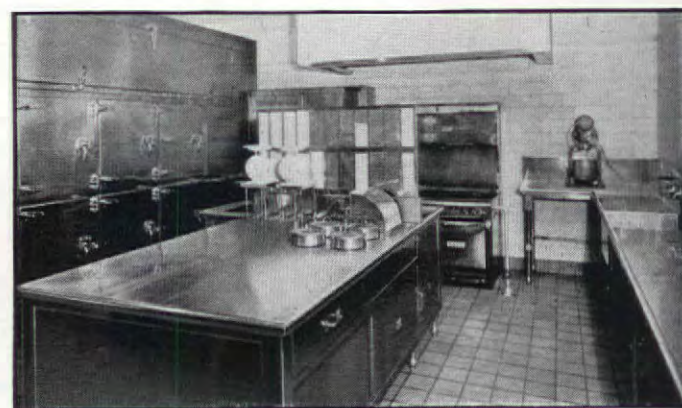
• Monel Metal food service equipment in special diet kitchen of the Kansas City General Hospital in Kansas City, Mo. Fabricated and installed by Duparquet Range Company of Chicago.
