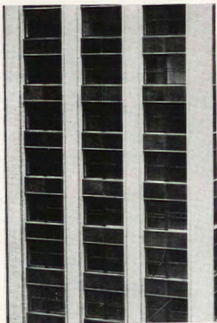
Close-up of Virginia Green Tremolite Spandrels, 280 Madison Avenue, N. Y., Walker & Gillette, Architects, N. Y.
