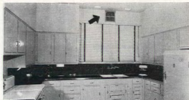
11g kitchen ventilating fan installed over window
