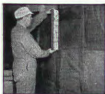
Gimco Sealal Bats fit standard spaced studdings. They can be obtained either with or without waterproofed paper backing.
