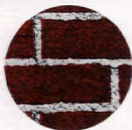
Actual photo of ordinary mortar joints. Note shrunken, cracked mortar, permitting rapid water seepage and destruction.
