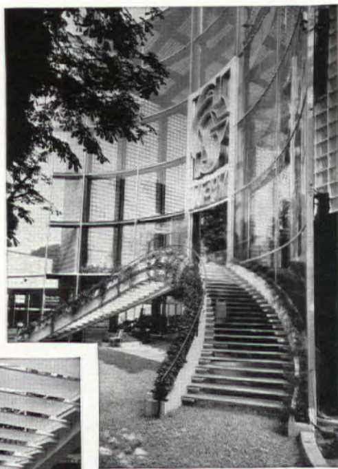
"THERMOLUX" GLASS MURAL , Italian Building, Paris Exposition. "Thermolux" is a European product consisting of glass cover plates between which is sandwiched a layer of glass threads, providing light diffusion and temperature insulation
