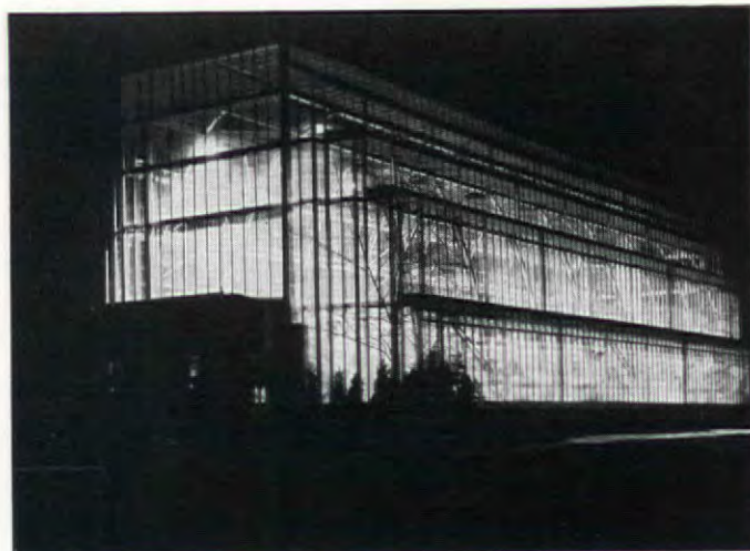
FLORAL CONSERVATORY , Forest Park, St. Louis. This structure contains 16,600 sq. ft. of double strength Libbey-Owens-Ford plate glass, is 186 ft. long, 55 ft. wide, and 55 ft. high. Glass panes are 24 by 26 in.
