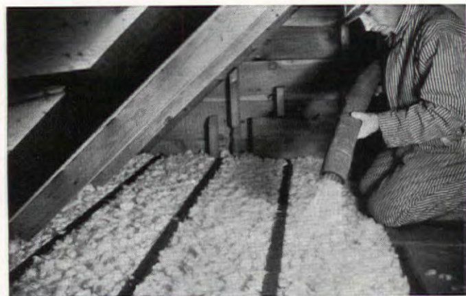
Nodulated glass fiber insulation is blown between joists and studs in the regular manner, particularly adapted to existing buildings
