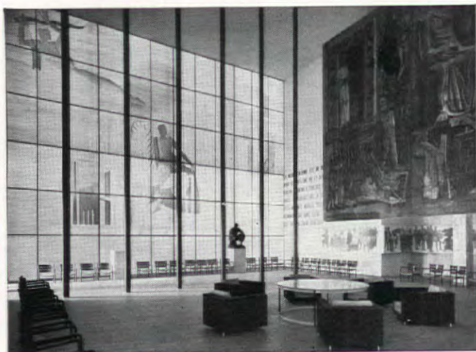
"THERMOLUX" GLASS MURAL , Italian Building, Paris Exposition. "Thermolux" is a European product consisting of glass cover plates between which is sandwiched a layer of glass threads, providing light diffusion and temperature insulation
