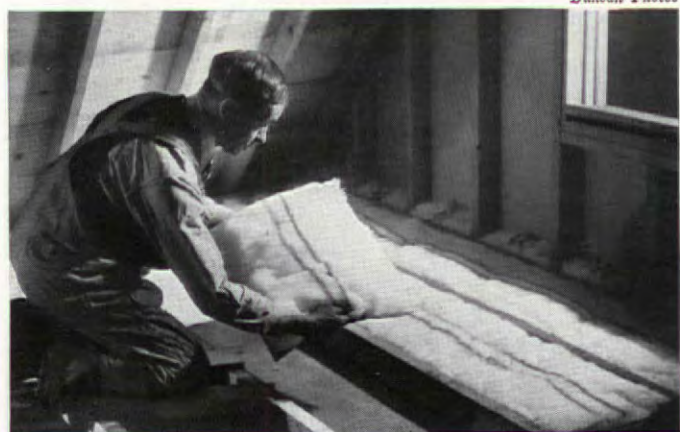
INSTALLATION of glass fiber insulation in "bat" form. Insulation shown in this picture and in the picture below made by the Owens-Illinois Glass Co., distributed by the United States Gypsum Co.
