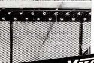
★ Standard Sheets of Metal Lath — applied without any previous wiring of channels to either Ceiling or Floor Runner. Tying completely done in one operation with ordinary tie wire. Here is a real saving in time.
