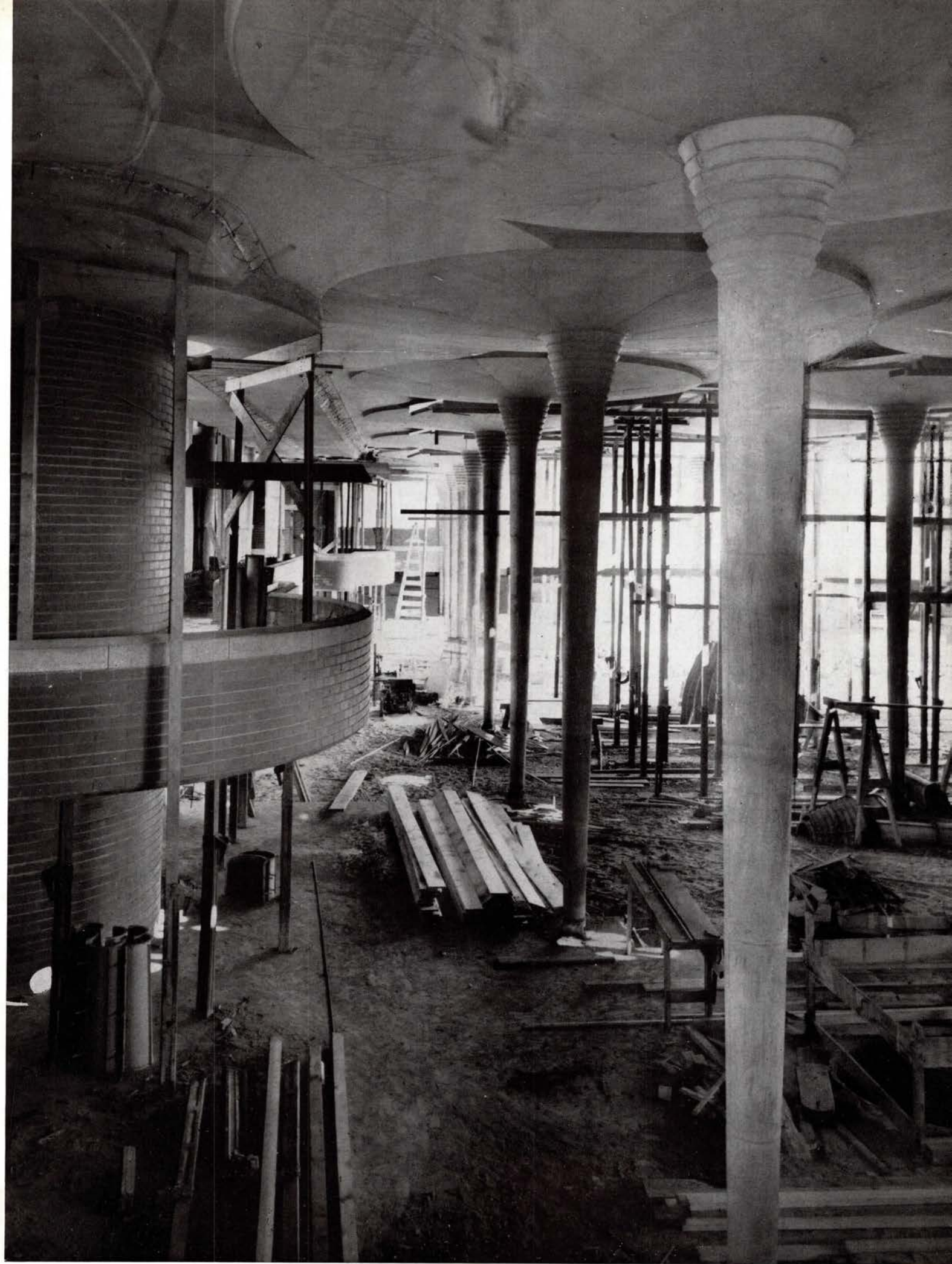
THE BUILDING IN CONSTRUCTION . ANOTHER INTERIOR VIEW OF THE BIG ROOM SHOWING DENDRIFORM COLONNADE . THE SENSE OF PHYSICAL WEIGHT DISSOLVED IN SPACE
