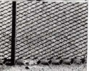
★ Slotted Channel Studs — notched at top for variations in ceiling heights. Slot slides over standing leg of Ceiling Angle Runner — bottom slips into place in grooves of Floor Runner. Metal lath tied to studs with tie wire.
