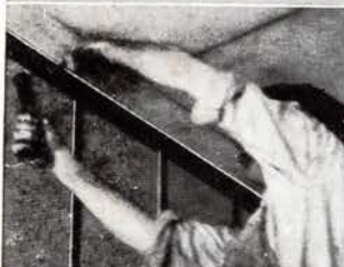
★ Ceiling Angle Runner — attached to ceiling with bolts, nails or Rawl Drives. Burr on holes prevents tipping of channels.
