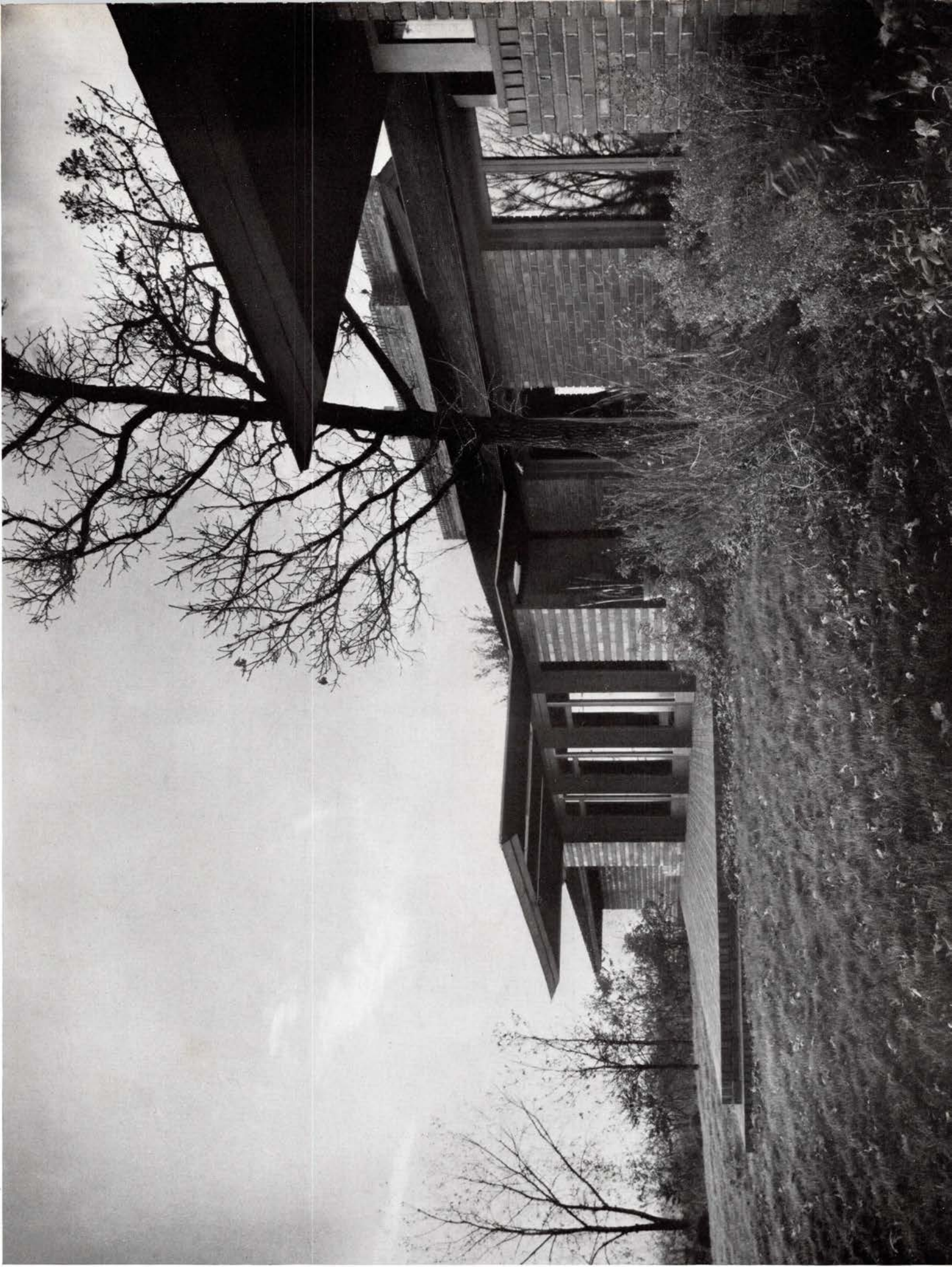
MALCOLM WILLEY HOUSE . . . VIEW FROM THE SOUTH . . . ALTERNATING LAYERS OF DARK RED SAND MOLD AND PAVING BRICK IN PAVEMENTS, WALLS AND FIREPLACE
