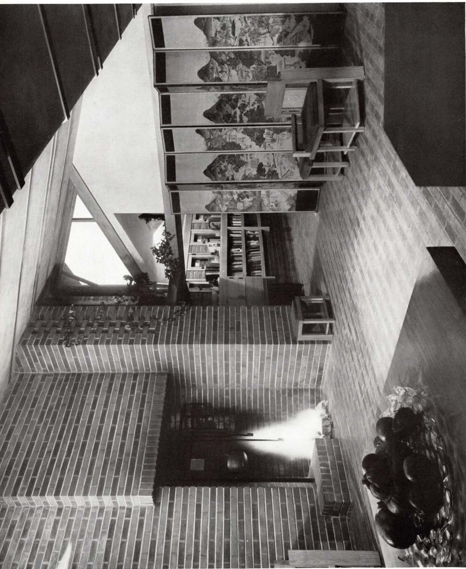
RED BRICK FIREPLACE IN LIVING ROOM OF MALCOLM WILLEY HOUSE . . . SAME ALTERNATING BRICK COURSES IN FLOORS AND WALLS . . . IRON CRANE AND INSERTED RED TILE
