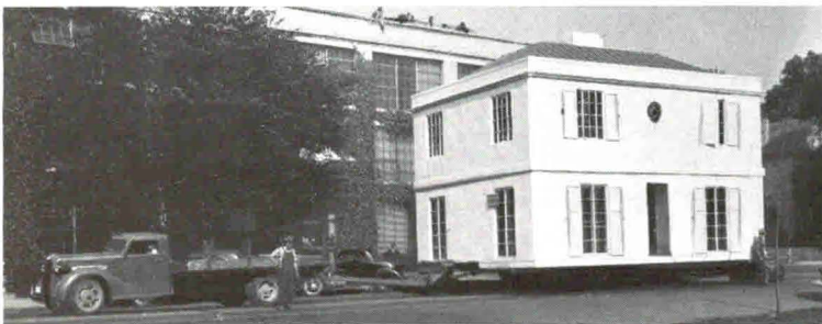
An arc-welded house on the way to its foundations. Plumbing is installed, walls painted, and shutters hung. The Hobart Bros. Co.
