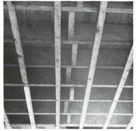
"SOLID BRIDGING BETWEEN FLOOR JOISTS. You are looking upward at the inner structure of the living room ceiling and second floor. Note the staggered bridging of solid, timber-width pieces spiked through the joists (center)."
