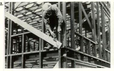
Stran-Steel Frame: 1. Bolting sill to foundation wall. 2. Diagonal bracing nailed directly to frame. 3. Setting wood window frames. 4. Placing pin in hinge connector for rafters.
