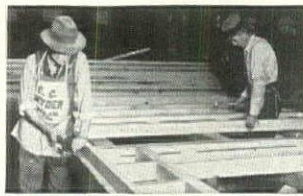
Precision-Built construction starts in the shop—where all lumber is pre-cut.
