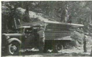
Complete sections are delivered by truck to the location.
