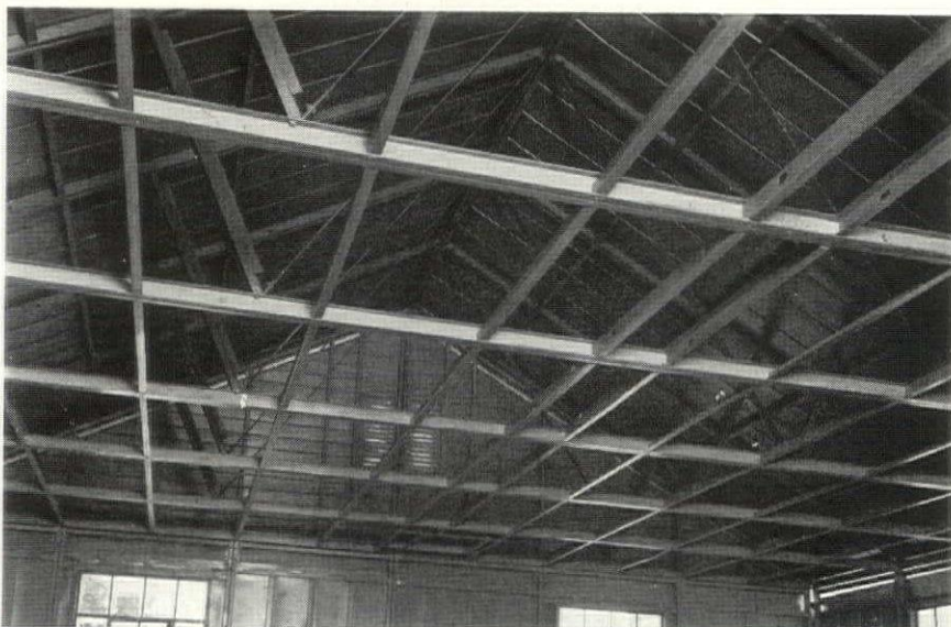
Construction view (above) shows steel ceiling joists and roof panels combined and reinforced to form rigid trusses. Note foundation, floor and wall construction in view, below.
