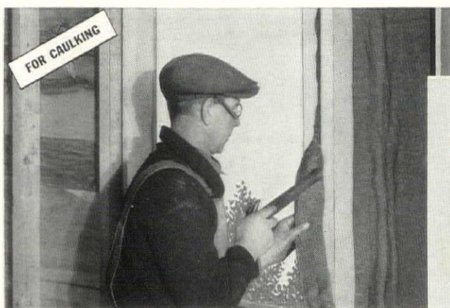
FOR SIDE WALLS AND ROOFS: Made in blankets of just the right width to fit snugly between studding, Kimsul minimizes fitting and cutting. In side walls simply nail one end of blanket to the header, draw the free end down and fasten at the bottom. In sloping roofs, the same easy procedure is followed, save that retaining laths are nailed along the edges.
