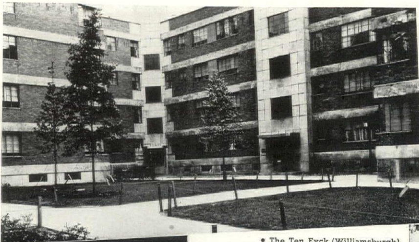
• The Ten Eyck (Williamsburgh) Housing Project. A 50,000-yard installation, of Milcor Solid Plaster Partitions in Buildings 1, 2, 3, 4, 6, 7, 8. Photo courtesy of FHA.
