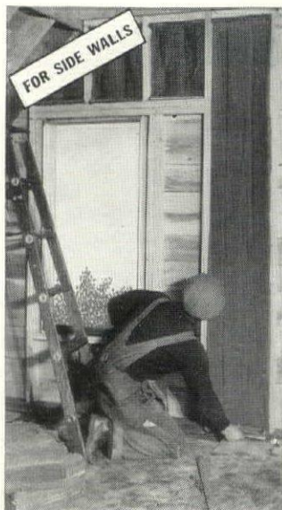
FOR SIDE WALLS AND ROOFS: Made in blankets of just the right width to fit snugly between studding, Kimsul minimizes fitting and cutting. In side walls simply nail one end of blanket to the header, draw the free end down and fasten at the bottom. In sloping roofs, the same easy procedure is followed, save that retaining laths are nailed along the edges.
