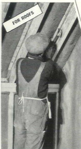
FOR SIDE WALLS AND ROOFS: Made in blankets of just the right width to fit snugly between studding, Kimsul minimizes fitting and cutting. In side walls simply nail one end of blanket to the header, draw the free end down and fasten at the bottom. In sloping roofs, the same easy procedure is followed, save that retaining laths are nailed along the edges.
