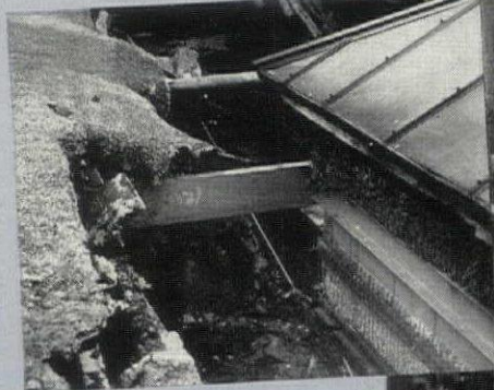
Costly lesson learned—the wood roof is being replaced by Firesafe GYPSTEEL PLANK.
