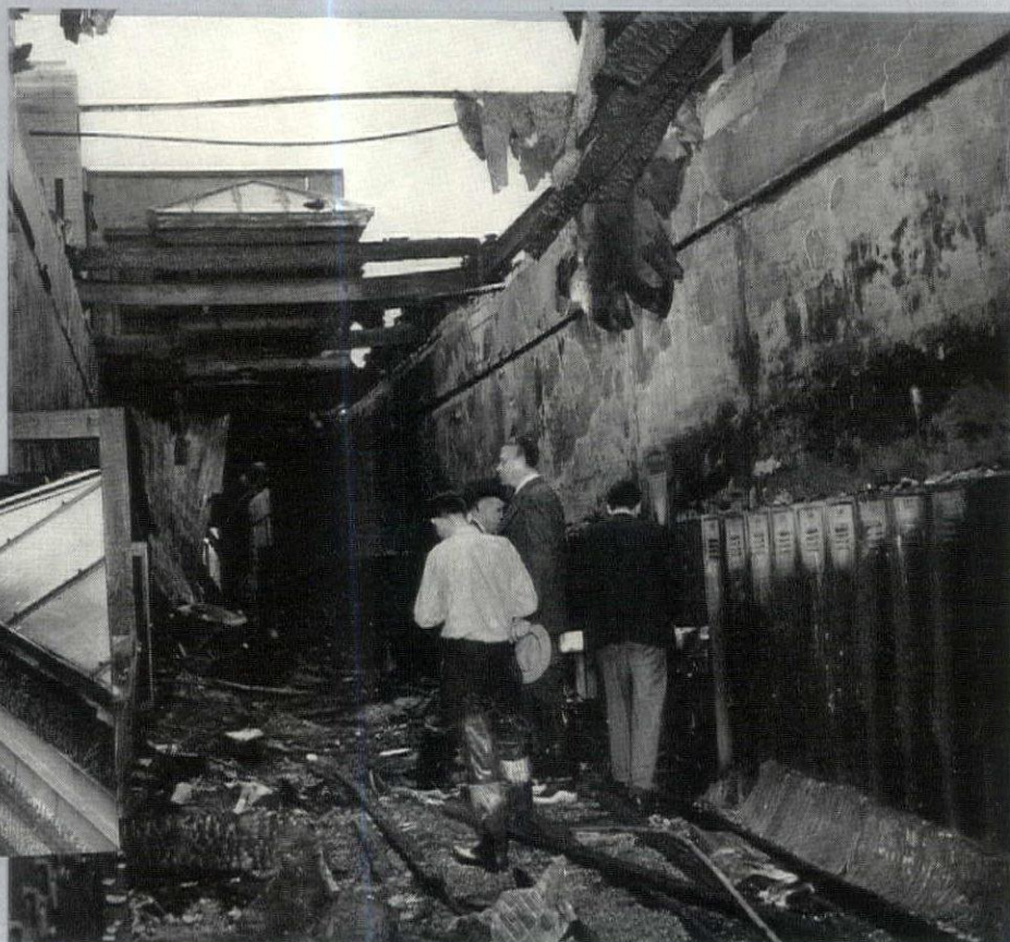
Costly lesson learned—the wood roof is being replaced by Firesafe GYPSTEEL PLANK.
