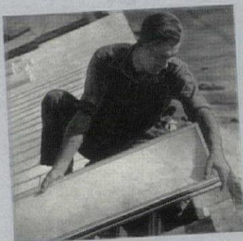
Costly lesson learned—the wood roof is being replaced by Firesafe GYPSTEEL PLANK.
