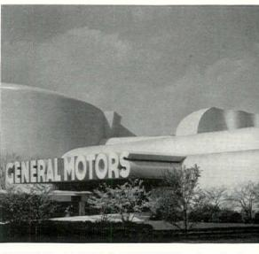
GENERAL MOTORS BUILDING — Actually four buildings centered around a cross street on which is staged a dramatic traffic show—in it you'll find 199,392 feet of SHEETROCK\*, and 201,712 feet of GYPLAP—used to help protect spectators against possible hazards of fire.
