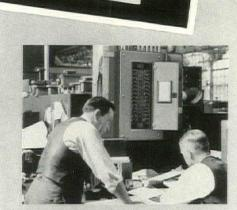
Nofuze panelboards give finger-tip control of electrical circuits — Safe, convenient, approved by Underwriters' Laboratories
