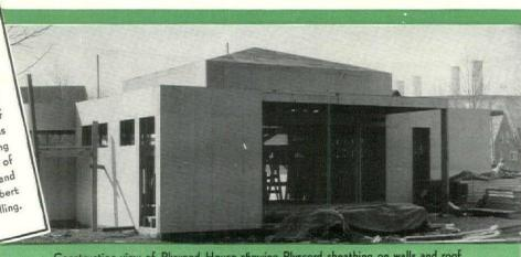
Construction view of Plywood House showing Plyscord sheathing on walls and roof.
