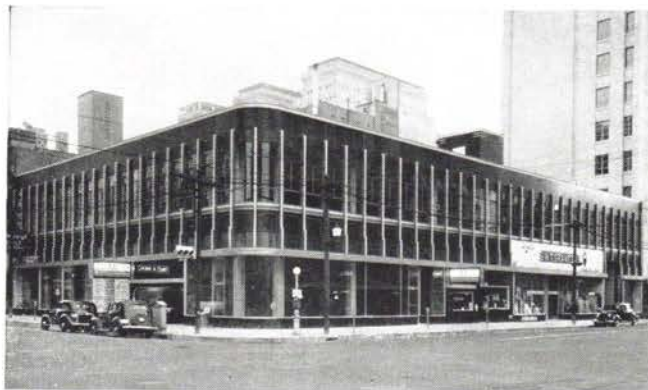
Polished Virginia Black Serpentine Facings and Bulkheads, Varner Bldg., Houston, Tex., Kenneth Franzheim, Archt.
