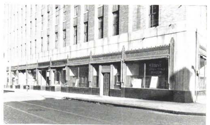
Polished Virginia Black Serpentine Bulkheads, United Shoe Machinery Co. Bldg., Boston, Mass.
