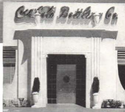
Main Picture: New Coca-Cola bottling plant in Waco, Texas. It's built with Architectural Concrete made with Universal Atlas Cement. Light green cement paint made with Atlas White cement on exterior. Sidewalks colored with green pigment. Architect, Robert V. Darrah, Los Angeles. Associate Architect, T. Brooks Pearson, Waco. General Contractor, C. C. Ramsey, Waco.
