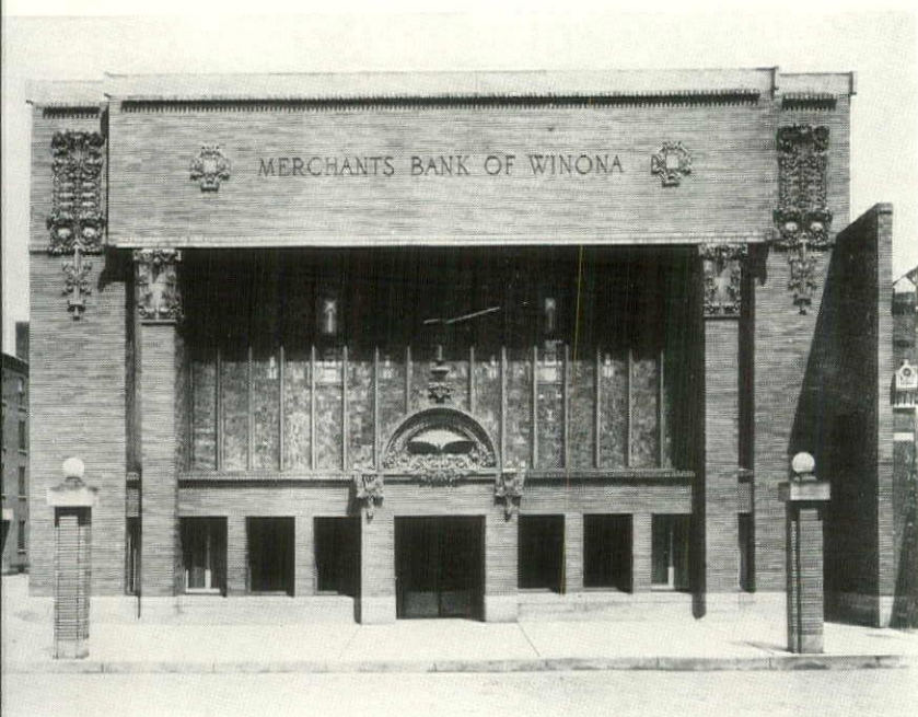
1912: Polychrome terra cotta with pale buckskin brick, Winona, Minn. Purcell, Frick & Elmslie, architects.
