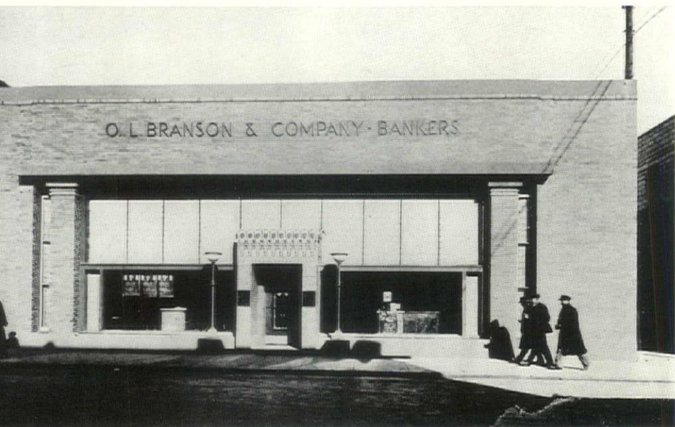
1916. A private banking house in Mitchell, S. D. For it Purcell & Elmslie designed an air conditioning system which, except for technical installations, must have been a pioneer.
