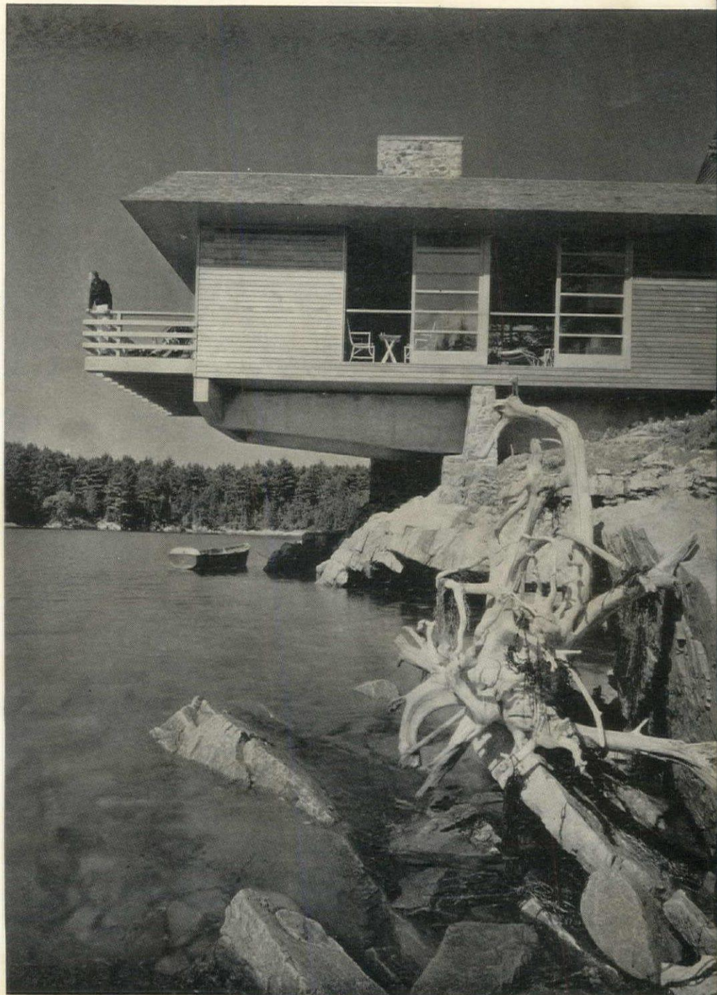
VIEW FROM EAST SHOWING LIVING ROOM ON CONCRETE CANTILEVER BEAM
