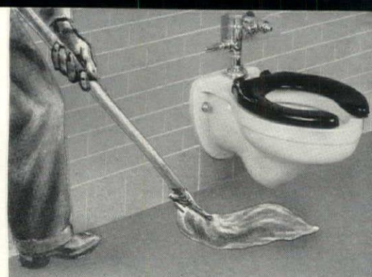
AID TO SANITATION. Wall fixture installations in toilet rooms and washrooms encourage cleanliness. Floors are easier to clean and keep clean.
