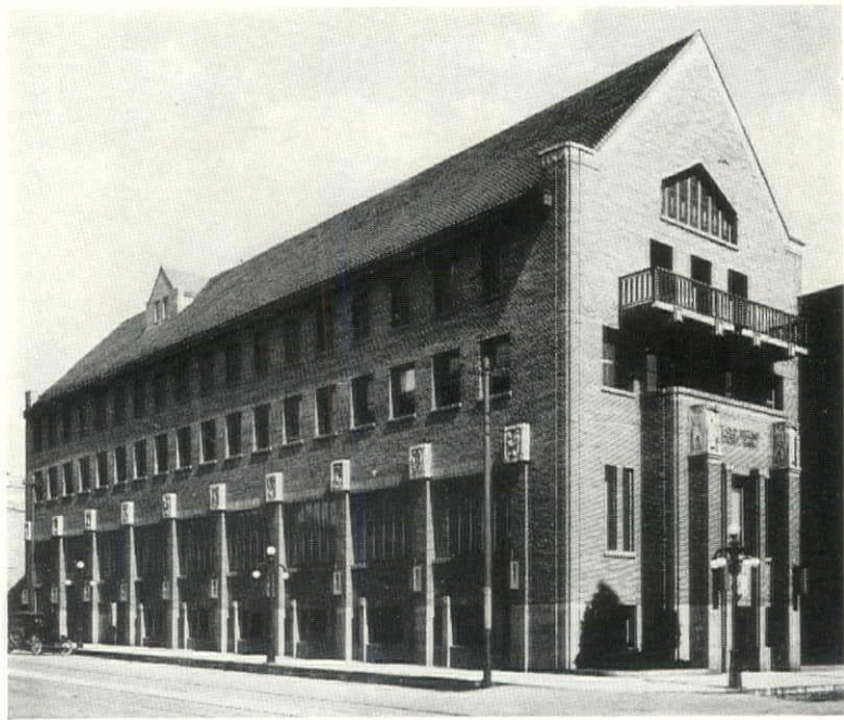
1924: The ends of reinforced concrete girders spanning banking room are sculpturally emphasized. Second National, Aurora, Ill. George Grant Elmslie, architect.
