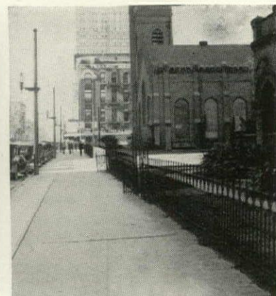
★ Sidewalk in Houston, Texas. Uvalde Rock Asphalt mastic laid in 1902—no repairs to date.
