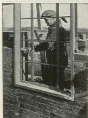
Easily installed . . . Casement and Casing slide down from top of wall; seated firmly in mortar at sill.
