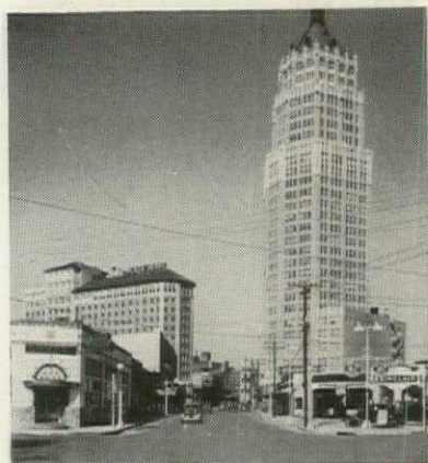
★ St. Marys Street, San Antonio, Texas. 3" Uvalde Rock Asphalt on a concrete base. No repairs to date after 22 years' service.
