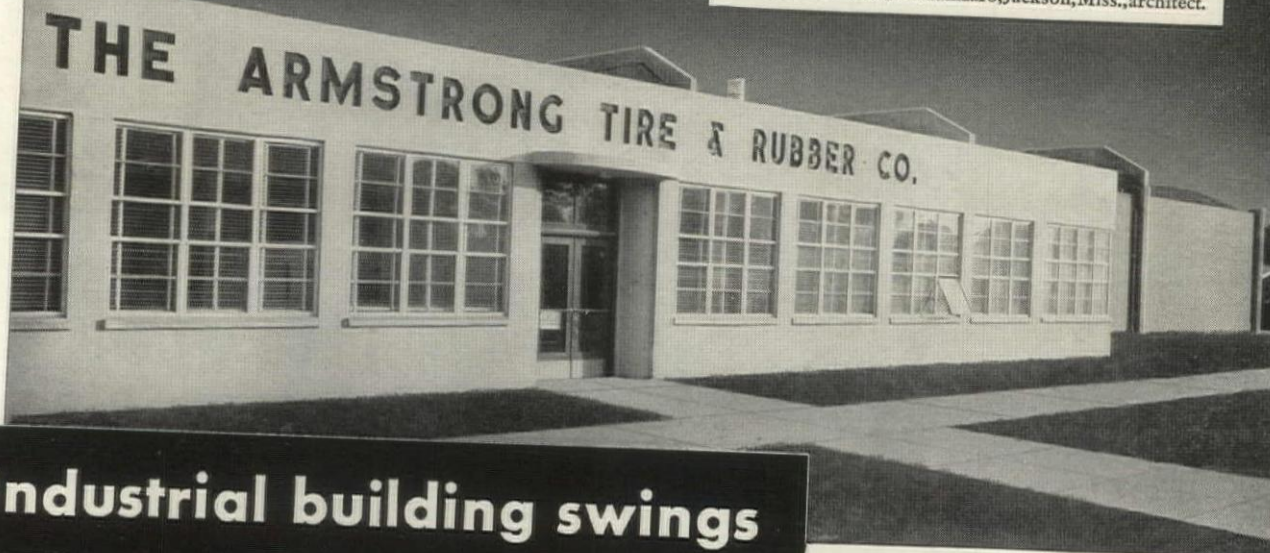
Armstrong Tire & Rubber Co. plant, Natchez, Miss. Main factory, 160 x 760 ft., office building, power plant. Architectural Concrete exterior walls; reinforced concrete Z-D barrel shell roof. Cost was very low. Roberts & Schaefer Co., Chicago, engineers, J. T. Canizaro, Jackson, Miss., architect.
