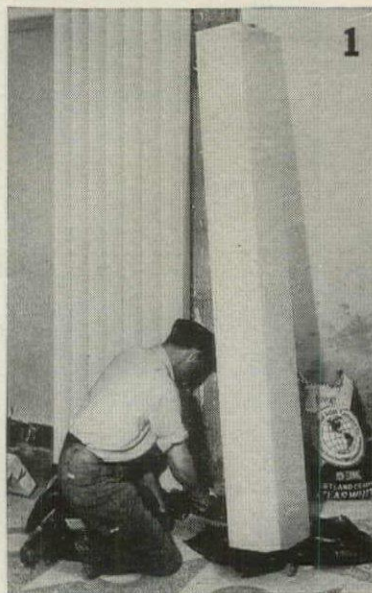
The David W. Taylor Model (Ship-Testing) Basin of U. S. Navy, Carderock, Md. Architectural Concrete Slabs were used as the outer forms for the structural concrete. An excellent bond was obtained, and half of the slab thickness was assumed as effective structurally. Designed by Rear-Admiral Ben Moreell, U. S. Navy. Architectural Concrete Slabs for exterior walls made with crushed quartz and Atlas White cement by Dextone Co., New Haven. Consultant, John J. Earley, Washington, D. C. General Contractor, Turner Construction Co., New York.
