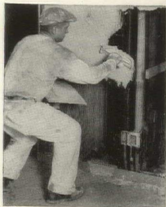
● 2 inches of solid plaster applied on standard Milcor Metal Lath.
