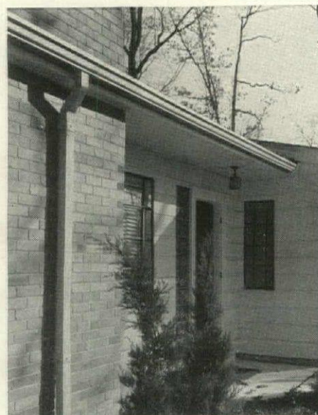
Home of W. P. Cole, St. Louis, Mo. Complete roof-drainage system of ARMCO Stainless Steel. Architect, Arthur B. Rathert, St. Louis.
