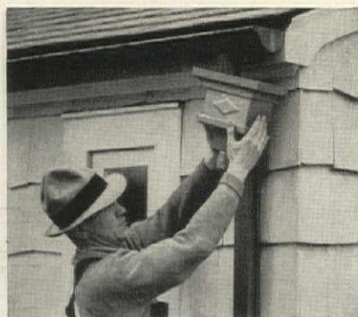
CHASE COPPER ROOFING PRODUCTS All Chase gutters, downspouts, heads, elbows, ridge rolls and flashings are full weight 16 ounce copper.
