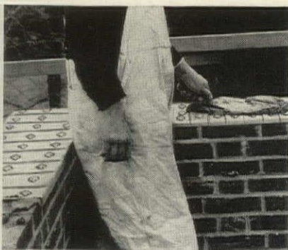
CHASE COPPER THRU-WALL FLASHING Directs water to face of wall. Helps to prevent masonry discoloration and inside wall leaks. Made of 16 oz. copper.
