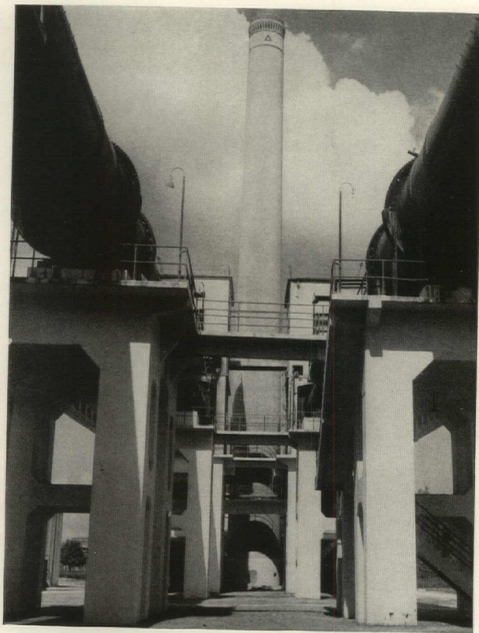
Concrete stack and rotary-kiln supports at one of Lone Star's plants.
