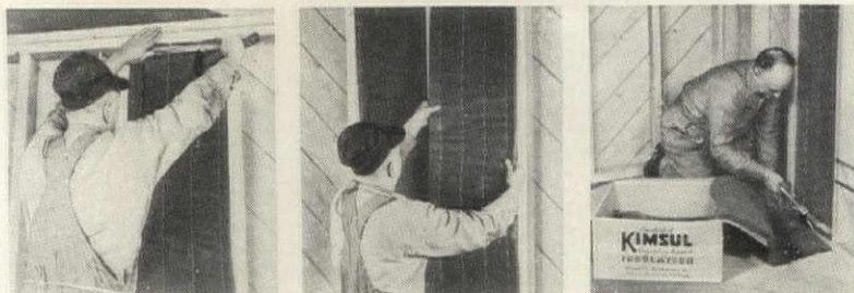
1. Attached to top plate with lath and nails . . . 2. Exactly fits standard widths and spacing . . . 3. KIMSUL is nailed at bottom—cut off—that's all!
