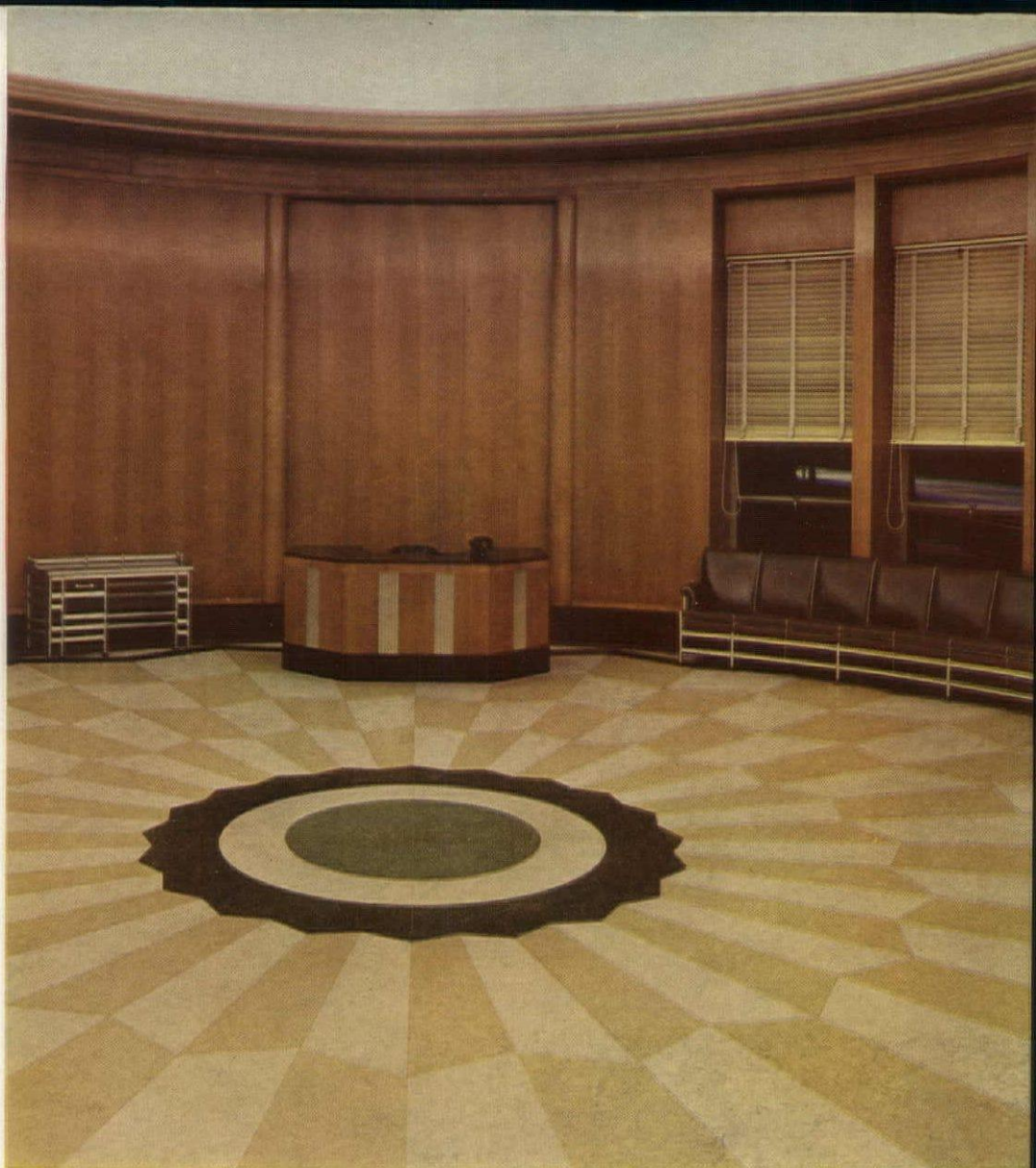
Terrazzo floor made with Atlas White cement in the Administration Building of the Chrysler Corporation, Detroit. Architect, Albert Kahn, Detroit. Terrazzo Contractor, Art Mosaic & Tile Company, Toledo.
