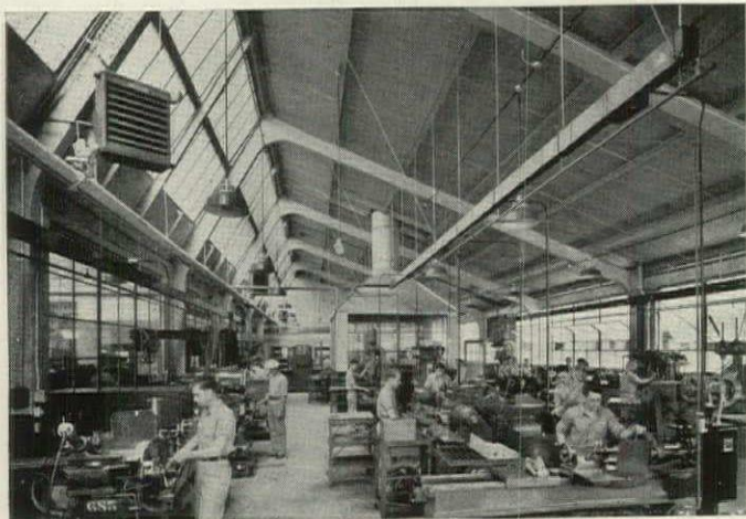
FACTORY design has long been conditioned primarily by daylighting requirements, with top-lighting, as in the above example by the Austin Co., a favorite solution. Sawtooth roofs are used where directional light is not objectionable, faced north to exclude sunlight, and monitors where light from opposite directions is a requirement.
