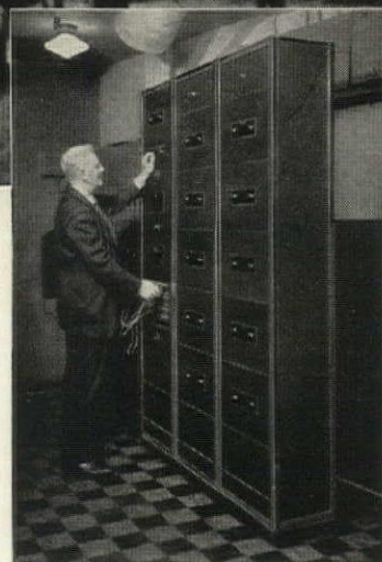
Complete Western Electric Sound Amplifying equipment for Madison Square Garden in New York City.
