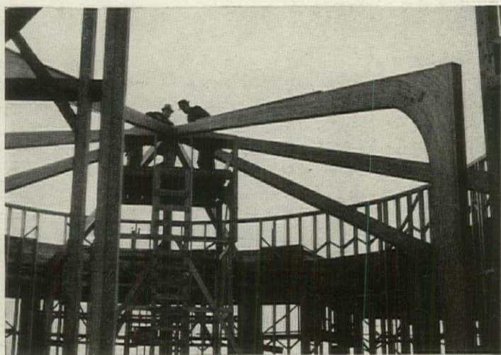
ERECTION of the eight completed arches was a simple matter of setting them on their bases and joining them together at the center with a hub. Arches support 48 ft. oval roof.
