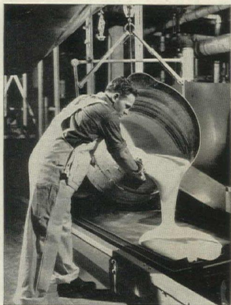
MANUFACTURE is by an entirely new process from liquid latex, the milk of the rubber tree, which is beaten into an air-filled froth, poured into molds, and baked. Upper pictures show native "milking" a tree, workman adding a jelling agent to beaten batch of latex, and operation of pouring an automobile seat cushion. Cores attached to the top of the mold form voids.
