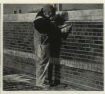
CHASE COPPER THRU-WALL FLASHING Directs water to face of wall. Helps to prevent masonry discoloration and inside wallleaks. Made of 16 oz. copper.
