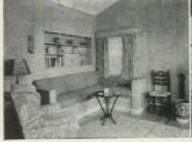
The walls of this attractive living room in Newport-Balboa, California, are 3/8" Plywall, are V-joined and lightly stained. The ceiling is Plyscord, painted. This combination was used effec-tively throughout the entire resused effecidence. Frank Green, architect.
