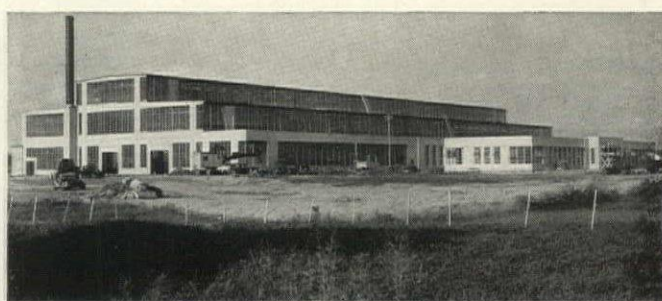
The plant of the Hydraulix Press Mfg. Co., Mt. Gilead, Ohio. Window and monitor areas are glazed with AKLO Hammered. Where large areas are exposed to the sun, AKLO greatly reduces heat infiltration.
