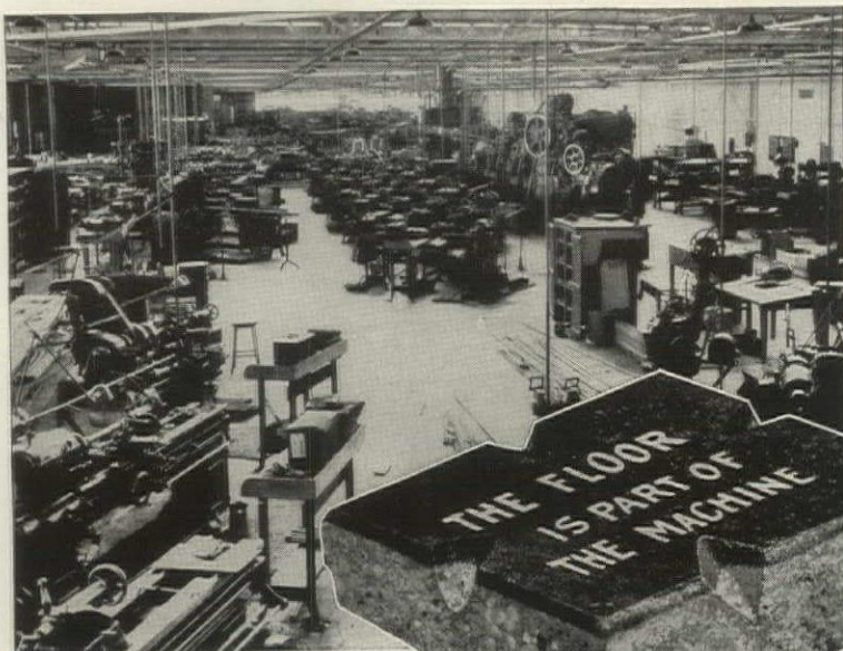
Note the great depth of metallic aggregate in this section of a Masterplate floor.
