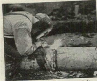
Welding conduit. With this connection, plain ring pipe supports are used and Conduit is free to slip over pipe, insulation and supports.
