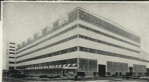
PHILA. NAVY YARD STRUCTURAL ASSEMBLY SHOP 68,000 sq. ft. White and Actinic C. W. G. Sidewall Construction
