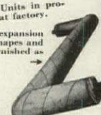
Shaker Square Co., Cleveland wrapping joint before installing connector.
