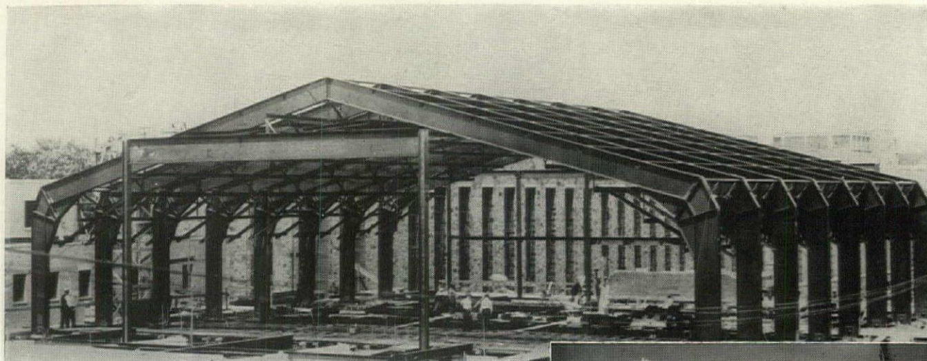
Welded Rigid Frames. (Photo courtesy of Schieve Construction Co., Buffalo)
