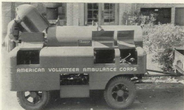
Portable unit built for American Volunteer Ambulance Corps—Sponsored by Dr. Alexis Carrel provides steam for sterilization—heating—cooking—and hot water needs. 25 HP., 125 lbs. pressure, length 12 ft., height 7 ft., width 6 ft., weight 6000 lbs. Insulation and steel lagging. Injector. Condensate recovery system. Fuel oil, cold and hot water tanks. Wash bowl—hot water and oil.
