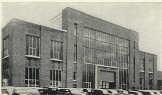
PHILA. NAVY YARD PIPE & COPPER SHOP 31,000 sq. ft. White and Actinic C. W. G. Sidewall Construction
