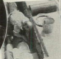
Shaker Square Co., Cleveland wrapping joint before installing connector.
