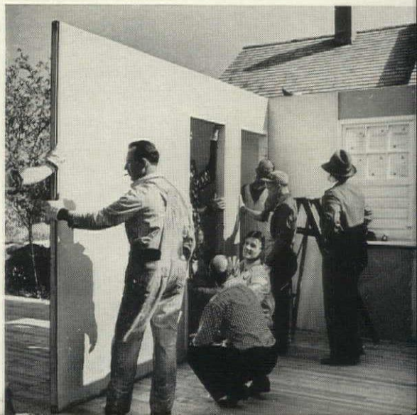
At eight o'clock Homasote's "junior" house takes shape as floor sections are anchored to piers laid night before (top). Half the rear wall, complete with windows, goes up as one piece, is set in floor clips, screwed to the smaller wall section (above). Note thickness of partition (below).
