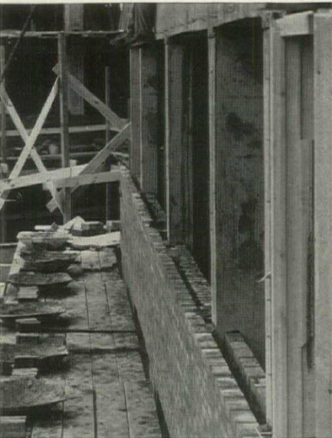
PANEL WALLS for this huge, concrete-frame apartment house in Montclair, N.J., designed by Sugarman & Berger, Architects, were built by the brick-cavity method. Photos
