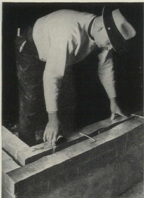
GOOD WORKMANSHIP is as necessary in cavity wall construction as in other forms of masonry. Pictures show mason placing damp-proofing at bottom of wall and successive
