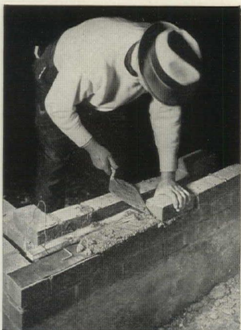
stages in use of wood strip to catch mortar drippings. Strip rests on wire ties placed in every sixth mortar joint to hold the "leaves" of the wall together, is pulled up with its
