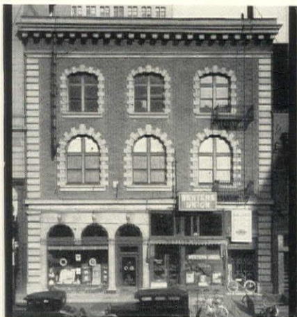
Removal of window arches, quoins and cornices and resurfacing with tile (first floor) and stucco brought the old George Building (13th, between Broadway and Franklin) up to date.
