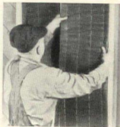
KIMSUL Quickly, Easily Installed Usually a one-man job. KIMSUL fits standard stud spacing, can be easily cut for narrow spacing, corners, etc.
