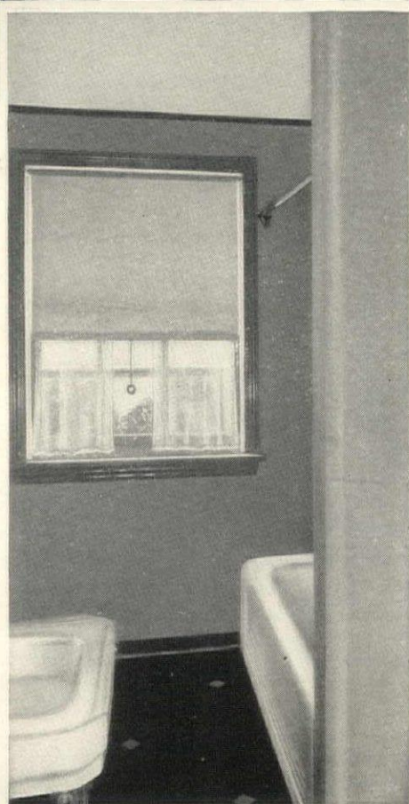
FRONT OF TUB RECESS in Mrs. Stearn's bathroom is a splendid example of how Nairn Wall Linoleum may be rounded to eliminate unsanitary cracks, give a more pleasing decorative treatment.
