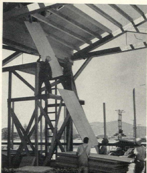
PLYSCORD roof sheathing (also used for walls and rough floors), roofs a defense plant in the northwest. Crew of 9, including 2 carpenters and 2 helpers, laid 32,000 sq. ft. in one 8-hour shift. A more experienced crew on a similar, simpler job, reported a labor cost of $2 per thousand feet. Plyform, another type of utility plywood for construction purposes, makes smoother concrete walls and permits multiple use of forms.
