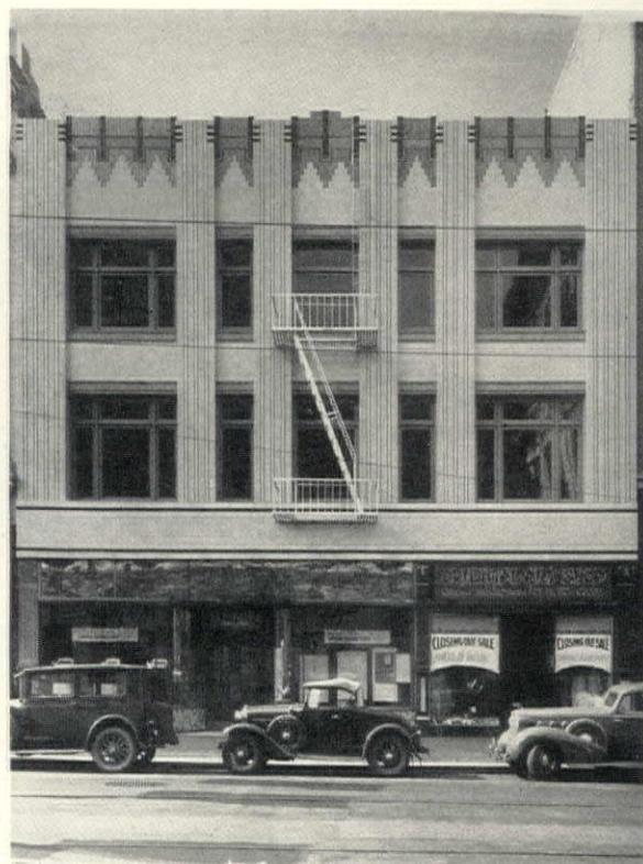
At a cost of only $4,580, the owners of the Fuller Building on 14th Street simplified the exterior of its top two stories, added a new fire-escape, helped offset the appearance of its untouched first floor.
