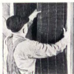
KIMSUL Quickly, Easily Installed Usually a one-man job. KIMSUL fits standard stud spacing, can be easily cut for narrow spacing, corners, etc.
